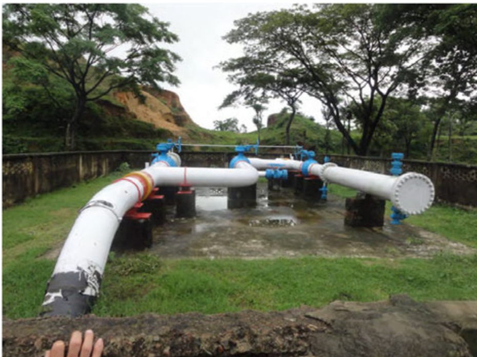
3) Shah mirpur manifold station (Tie-in point at East bank of Karnaphuli river)
