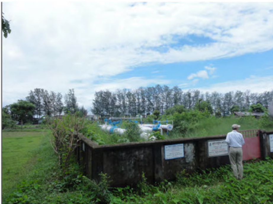
4) Patenga metering station (Tie-in point at West bank of Karnaphuli river)
