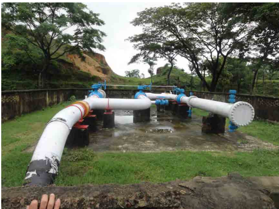
3) Shah mirpur manifold station (Tie-in point at East bank of Karnaphuli river)
