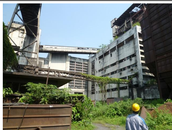
Site Survey in Existing Plant Area (Units No.4/5, Boiler Side)
