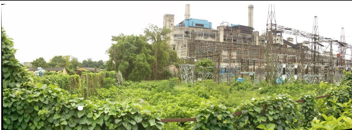
Switchyard of Units No.6/7
