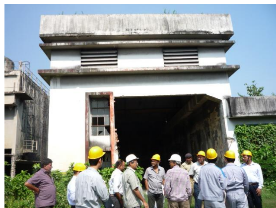
Site Survey in Existing Plant Area (Reuse: Circulating Water Pump House of Units No.1-3)
