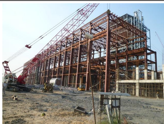
Construction of Units No.8/9 (Common Turbine Building)
