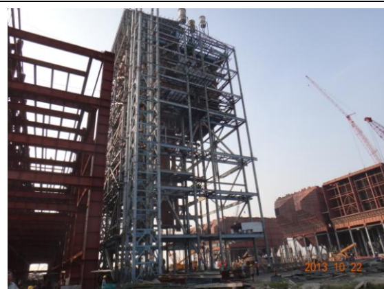
Construction of Units No.8/9 (Unit No.8 Boiler)
