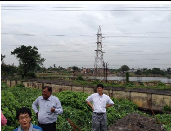
Transmission Line in north of Existing Plant
