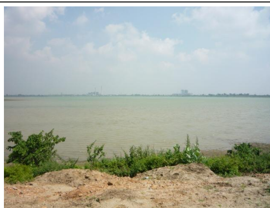
Inland Provisional Reservoir on Bank of the Ganges River (Barauni TPS in back)
