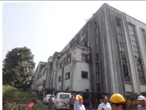
Site Survey in Existing Plant Area (Obsolete Turbine Building of Units No.1-3)
