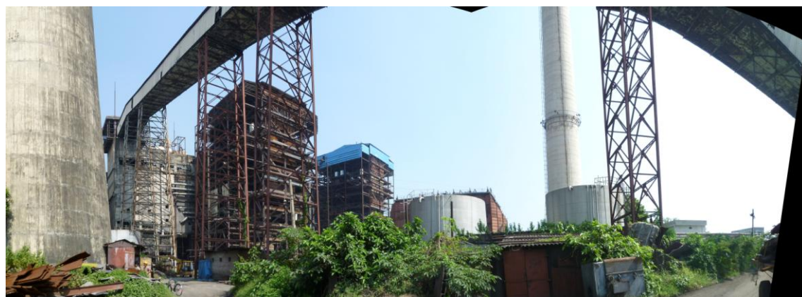
Site Survey in Existing Plant Area (Units No.6/7 under R&M/LE)
