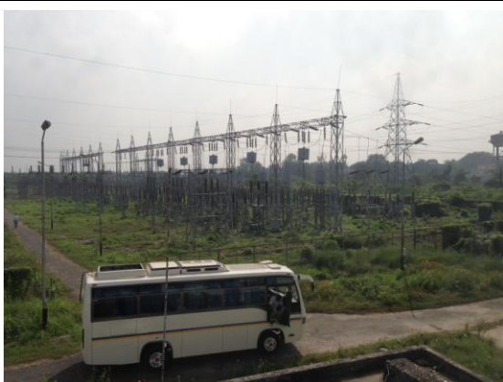
Visit Substation in north of Barauni TPS
