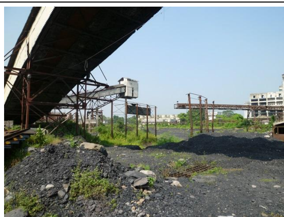
Site Survey in Existing Plant Area (Reuse: Coal Storage Yard)
