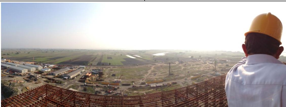
Site in the South adjacent to Units No.8/9 (from top of Unit No.8 Boiler)
