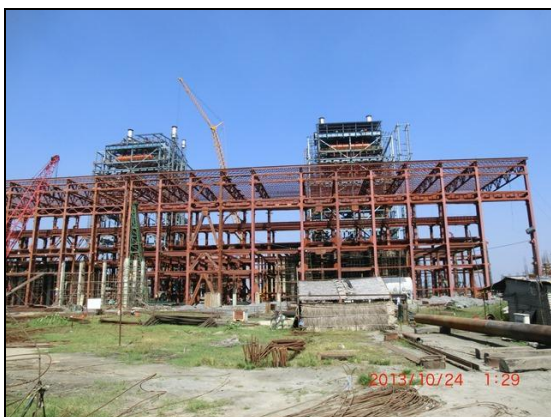
Figure 4.4-3 Units No.8/9 Construction Situation
