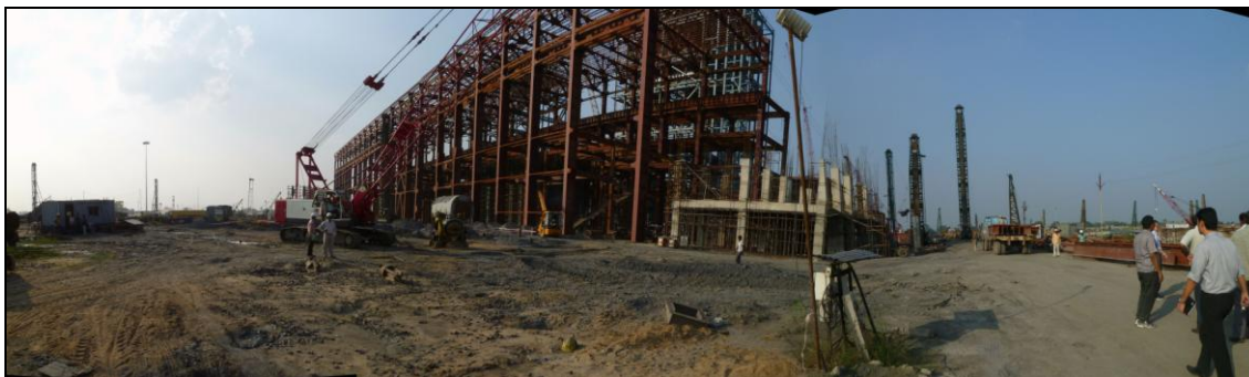
Figure 3.1-7 Construction of Units No.8/9 (Turbine Building)
