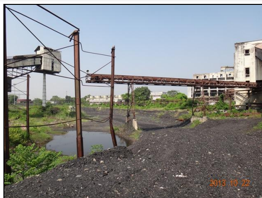
Coal Storage Yard
