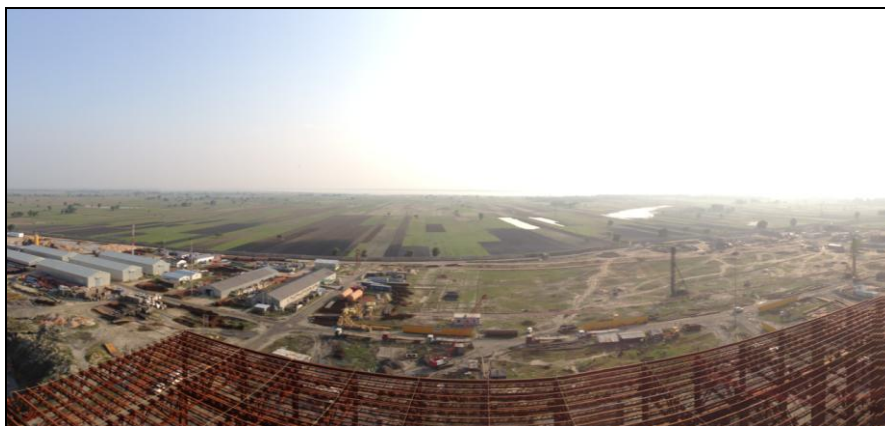
Figure 4.2-8 Site in the South Adjacent to Units No.8/9 (View from the top of Unit No.8 Boiler)
