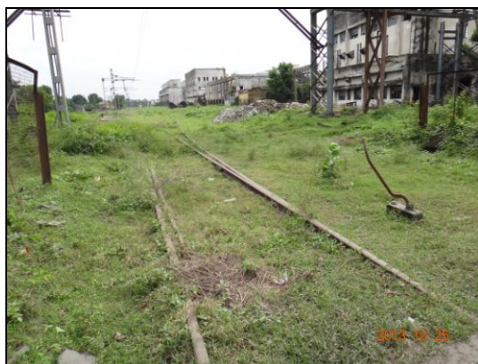
Existing Railway Track
