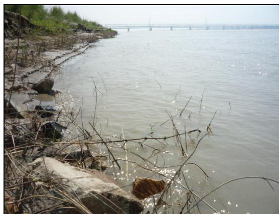
Figure 4.5-2 Left Bank of the Ganges (Downstream Side of Water Intake Point)
