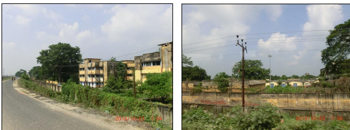
Figure 4.2-5 Situation in the Building of Residential Area
