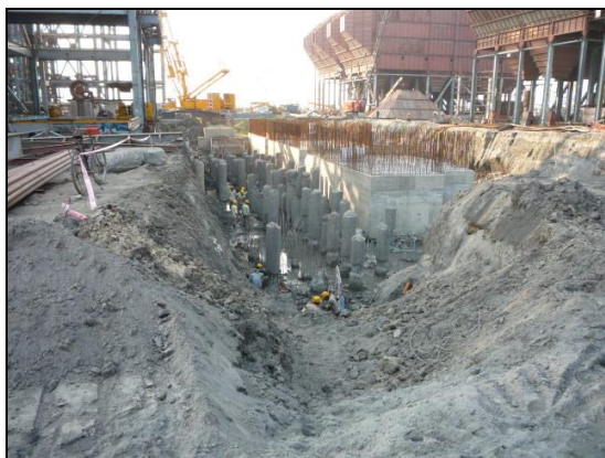
Figure 4.4-5 Bunker of Pulverizer Pile Foundation Construction
