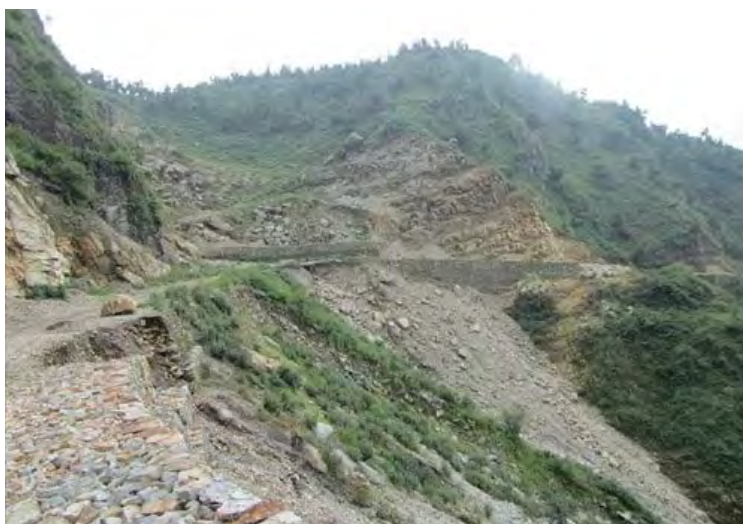
Figure 6.8.2 Site Photograph showing Slope Failure
