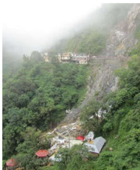
Source: JICA Preparatory Survey Team Figure.2.1.2 Slope Failure Distributed in the Sightseeing Area
