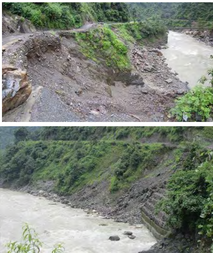
Figure 2.1.4 Road Shoulder Failure Occurred along the River (Rajbala Road in Dhalin in Kalsi Forest Division)
