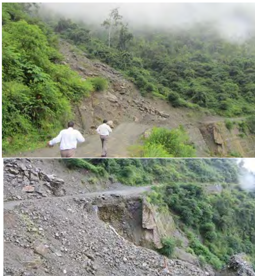
Figure 2.1.3 Slope Failure in Concave Landform
