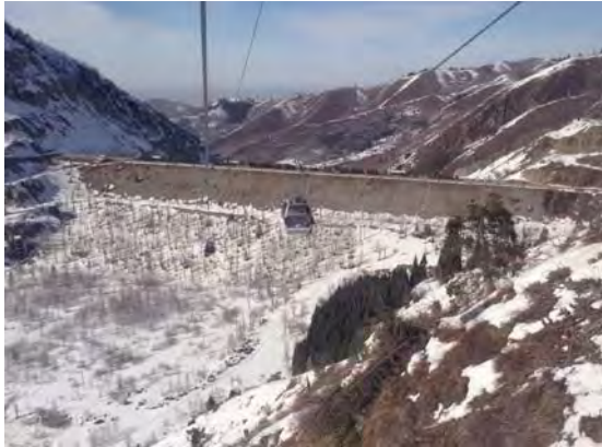
Medeu Dam (from upstream side) (H=250m, completed in 1973)
