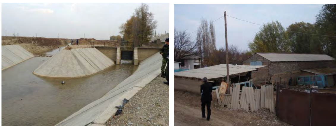
(Left: bank protection and small weirs, Right: a house affected by the flood)
