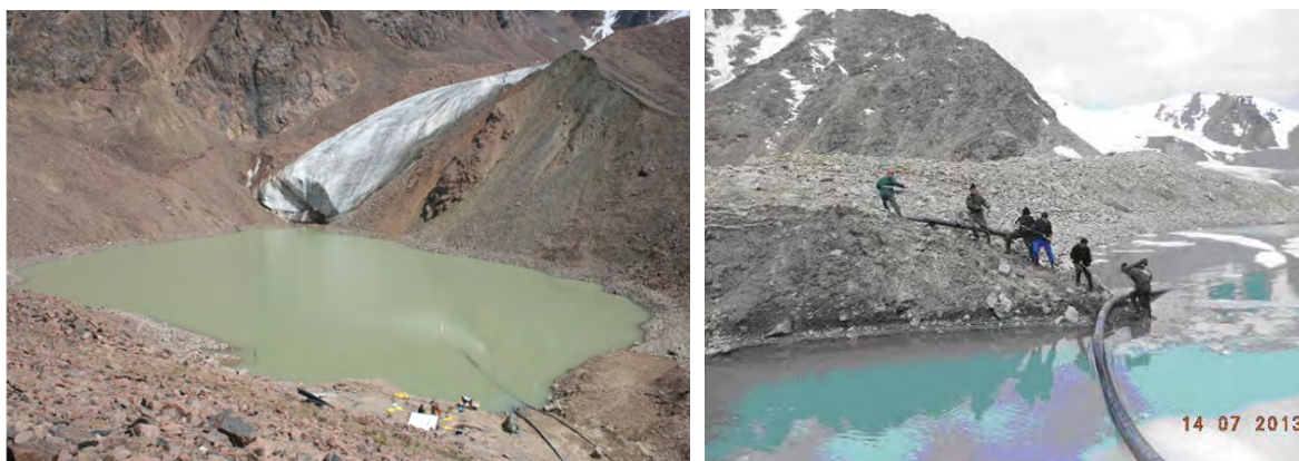
Figure 10.2 Adjustment of Water Level of Glacier Lakes Using Water Pipes
