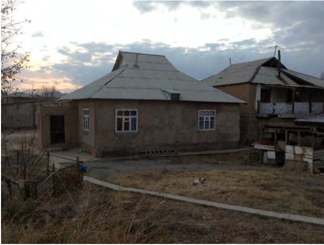
Many houses made of mud wall in the suburbs of Simkent are vulnerable to earthquakes or floods. (November 18, 2013, Shimkent)
