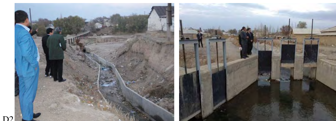
(Construction of drainage channel and floodgates)
