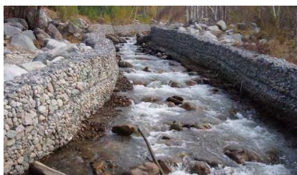
Figure 10.7 Channel Protection with Gabions
