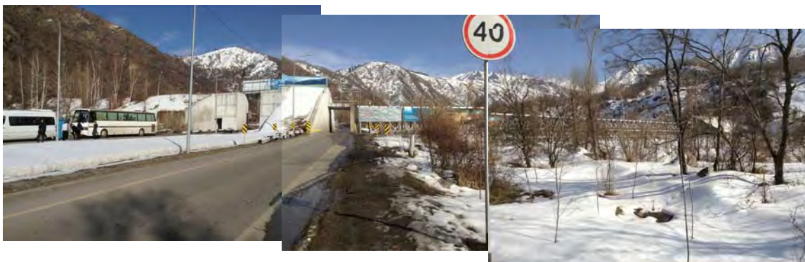
Steel Slit Dam (from downstream side)
