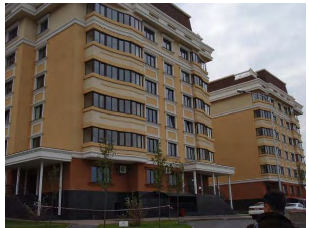
The project of Korkem Tau Residential Complex using Japanese aseismic technology (November 2, 2013, Almaty)
