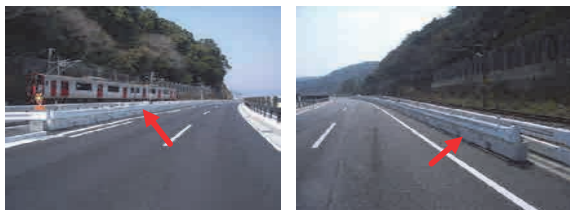
Installation of movable guard rail
