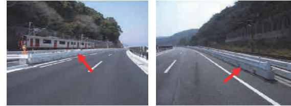
Installation of movable guard rail
