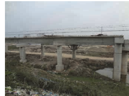
Flyover under Construction
