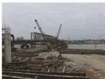
photo3-1(Ninh Binh bridge)
