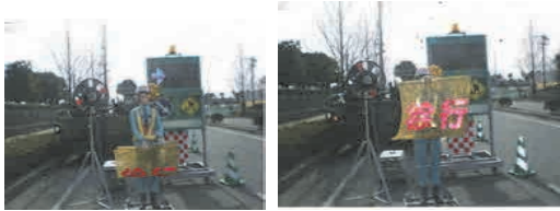
Installation of traffic control robot
