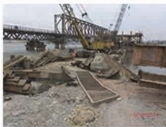
photo3-17(Way to barge)
