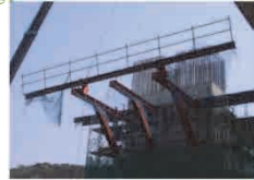
Pre-installation of handrail
