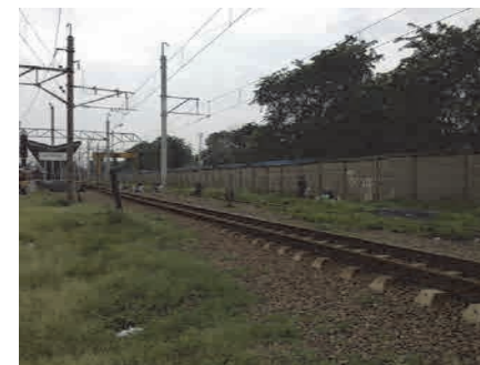
Bekasi Station - Railway
