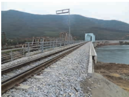
Track from the Right Bank (HCM Side)
