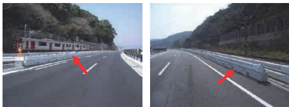
Installation of movable guard rail
