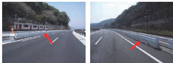
Installation of movable guard rail
