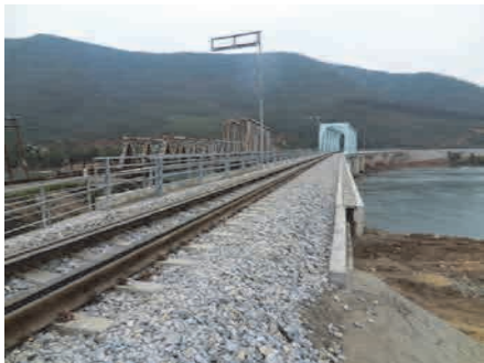
Track from the Right Bank (HCM Side)
