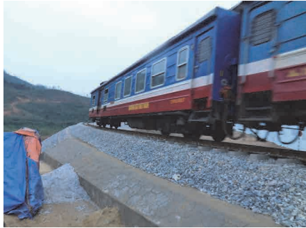
Track Vicinity Work at the Left Bank
