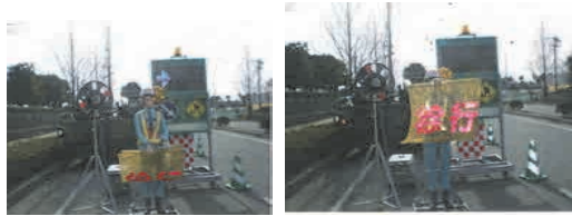
Installation of traffic control robot
