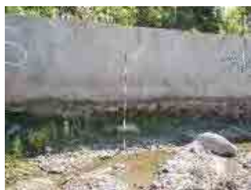
護岸前面の洗掘
