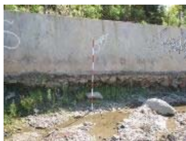
護岸前面の洗掘
