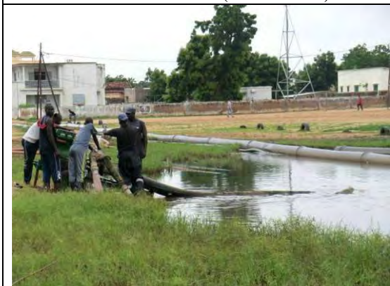
Drainage by Mobile Pump
