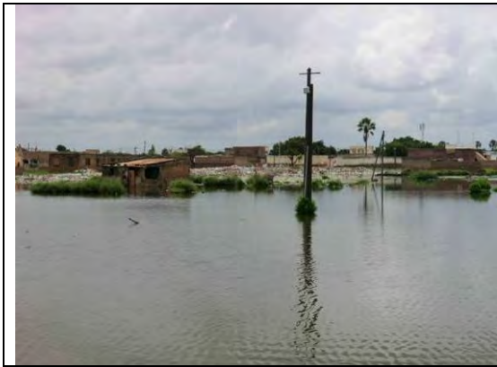
Inundation Condition (Lowland Area)
