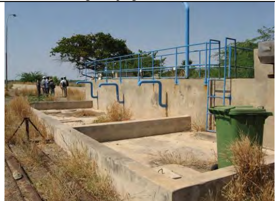
Sewage Treatment Plant (Grit Chamber)
