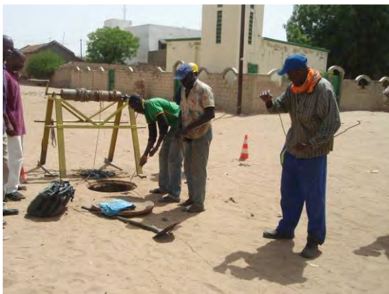
PHOTO 2.2.2 MANUAL CLEANING WORK WITH BRUSH
