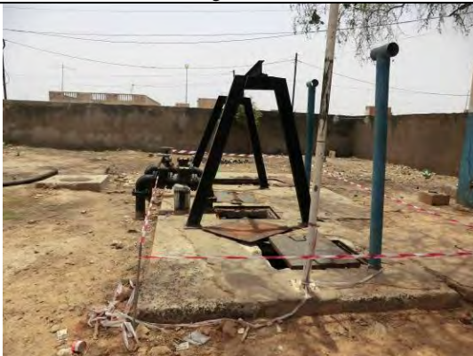
Existing Pumping Station (PS No. 3)
