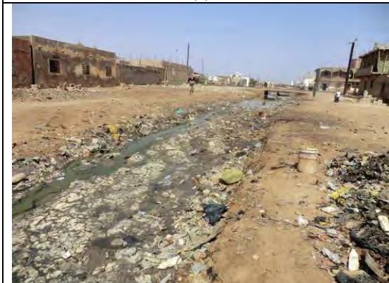
Excavated Earth Canal
