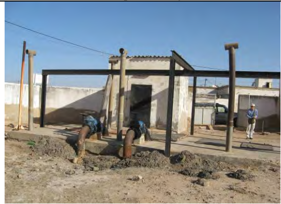
Existing Pumping Station (PS No. 2)
