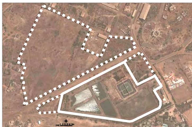
Fig. 4.3.1 Existing STP and Proposed Expansion Area
