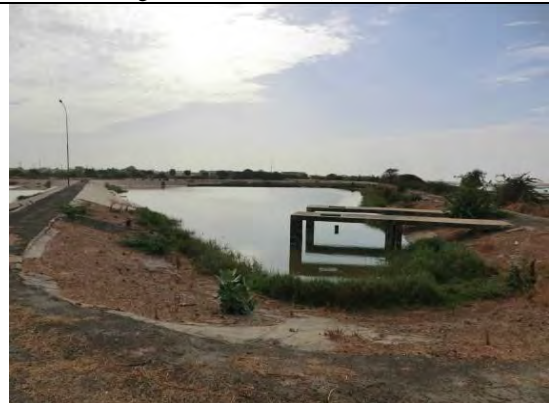
Sewage Treatment Plant (Maturation Lagoon)
