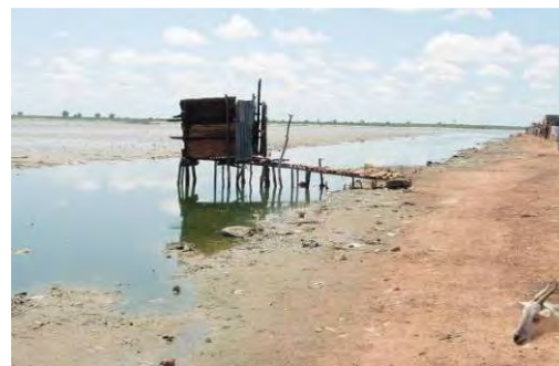
Toilet is located on muddy flat so that excreta is disposed directly to the environment (in Abattoirs District)
