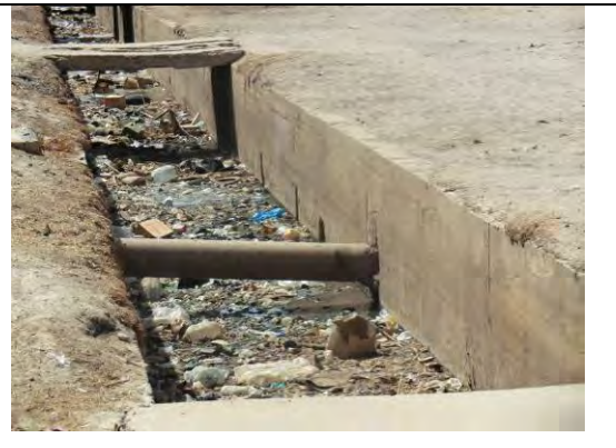
Obstacles in Open Drain
