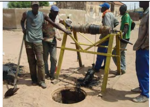
Manual Pipe Cleaning Work
