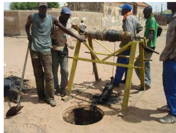
PHOTO 2.2.2 MANUAL CLEANING WORK WITH BRUSH
