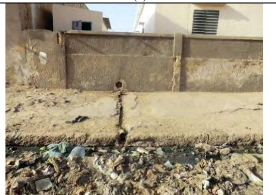
Sewer Pipe from Residence to Drainage Ditch
