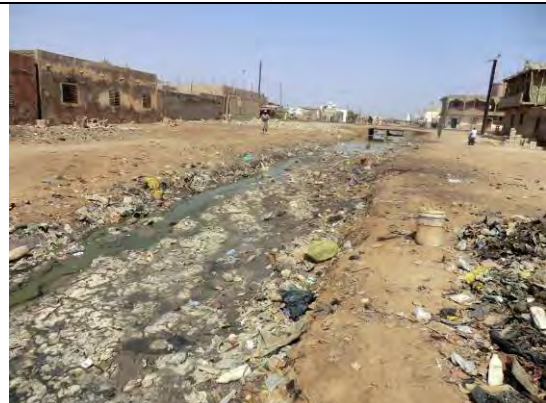
Excavated Earth Canal
