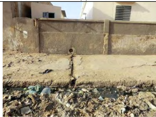
Sewer Pipe from Residence to Drainage Ditch
