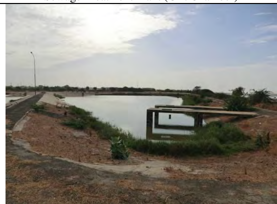
Sewage Treatment Plant (Maturation Lagoon)
