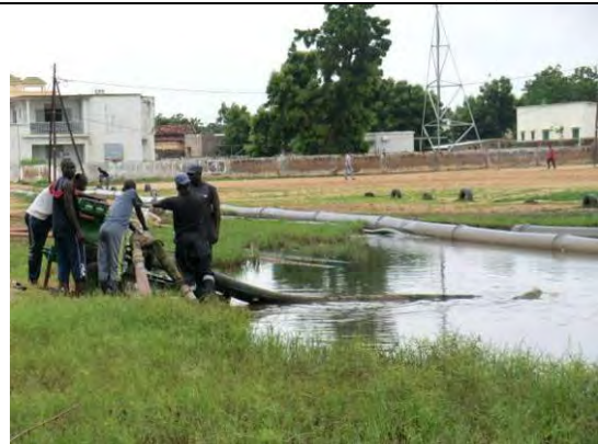
Drainage by Mobile Pump
