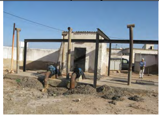
Existing Pumping Station (PS No. 2)
