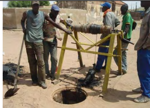
Manual Pipe Cleaning Work
