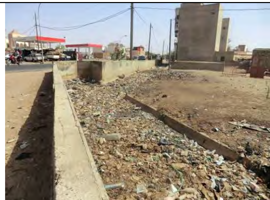
Illegal Dumping of Solid Waste and Sediment in Drain (2)
