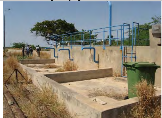
Sewage Treatment Plant (Grit Chamber)
