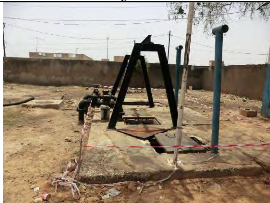
Existing Pumping Station (PS No. 3)
