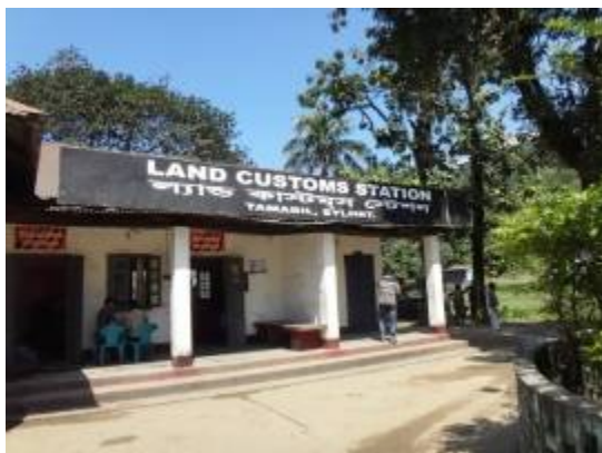
Bangladesh – Tamabil Land Customs Facility
