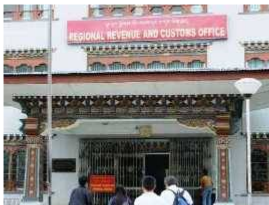
Bhutan – Regional Revenue and Customs Office, Phuentsholing
