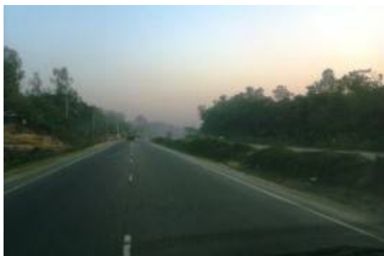
Bangladesh – Road N1 (Chittagong–Baraiyarhat)
