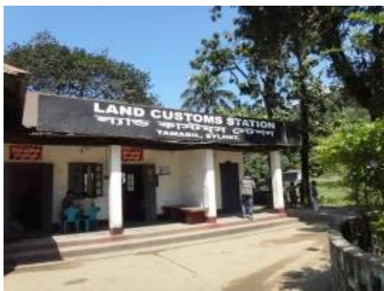
Bangladesh – Tamabil Land Customs Facility
