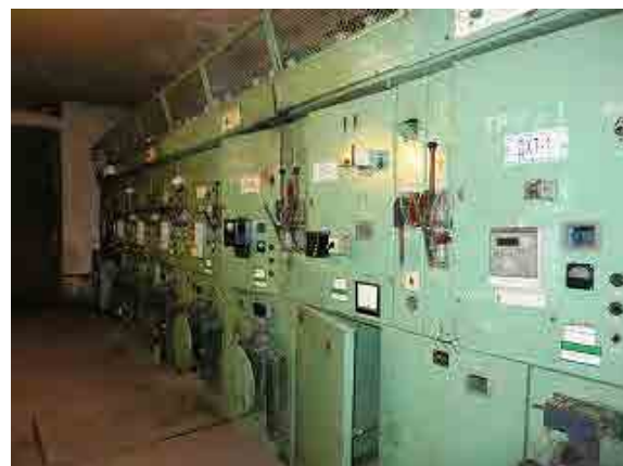
Figure 5-11 Circuit Breakers
