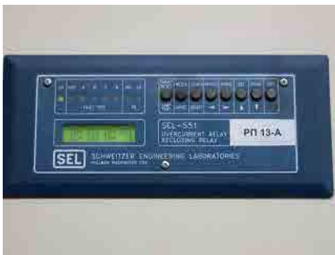
Figure 5-7 Protective Relay (Manufactured by SEL (USA))(Some of these relays have DGR. -40 degree Celsius specification 10 year guarantee)
