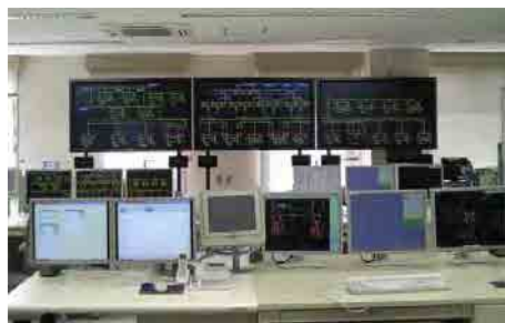
Figure 8-10 Image of the Supervisory Remote Control Device (Monitor)
