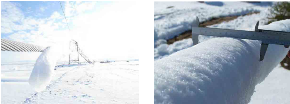
Figure 4-12 Tower Collapse Accident due to Ice & Snow Accretion
