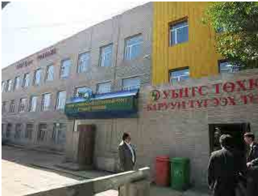
Figure 5-26 Distribution Center in Western Area
