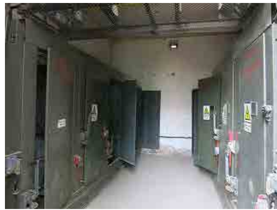
Figure 5-13 Load breakers (A system/B system)
