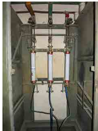
Figure 5-15 Transformation Protection Fuse
