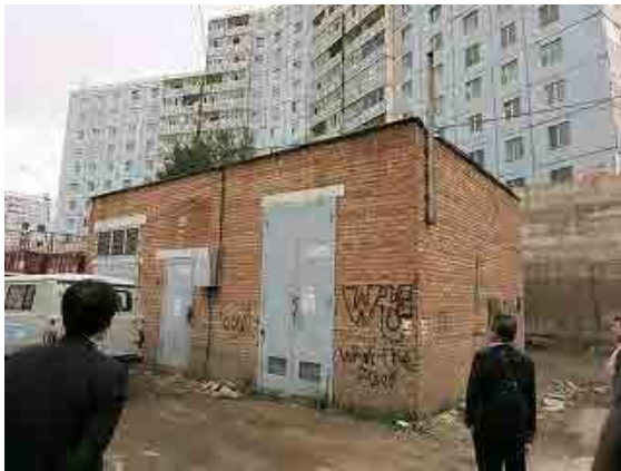
Figure 5-12 Exterior of Distribution Transformer
