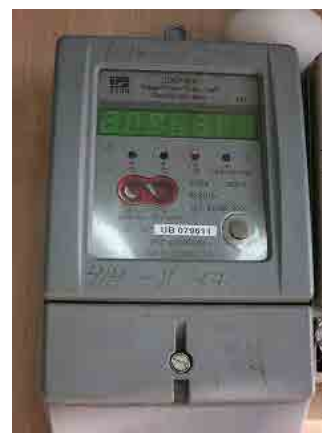
Figure 5-30 Meter for Time of Use(1 phase 2 wires)
