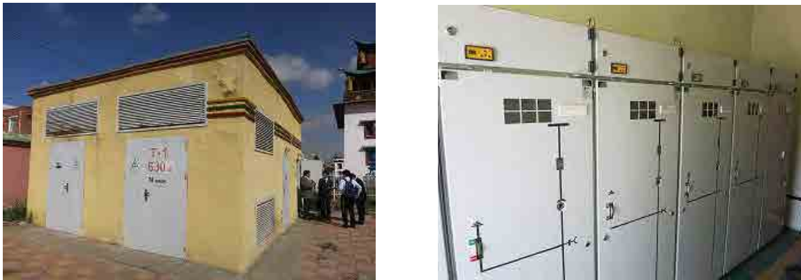
Figure 5-17 Distribution Transformer with Ring Main Unit (RMU)
