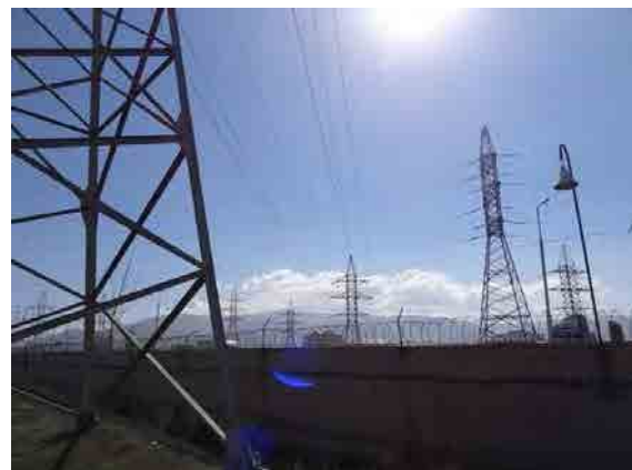
Crossing of 220kV T/L (No.1~No.2)
