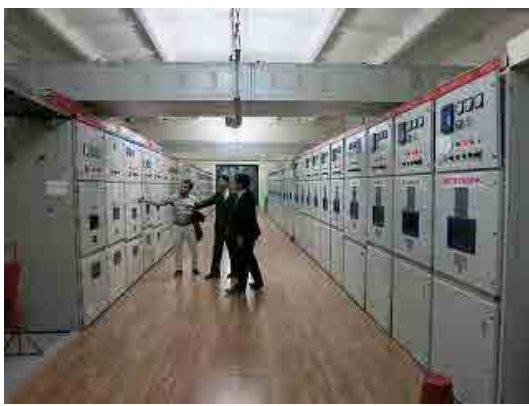
Figure 5-6 Inside of Substation and Distributing Circuit Breaker (Made in China. Right: 10kV, Left: 6kV. There are some heaters.)
