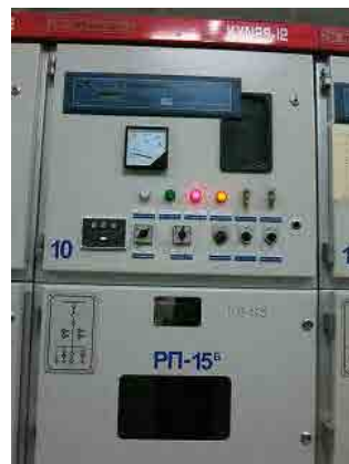
Figure 5-6 Inside of Substation and Distributing Circuit Breaker (Made in China. Right: 10kV, Left: 6kV. There are some heaters.)
