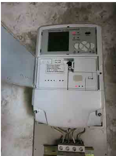
Collector with 3G in the distribution transformer
