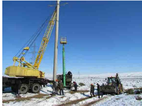
Repair Work on a Transmission Line Accident
