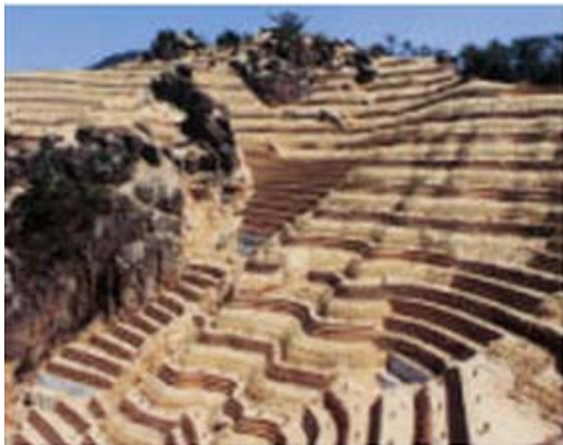
Terrace Making by local woods for Afforestation at Tanakami Mt, Shiga Source: Yodogawa River Office MLIT, HP
