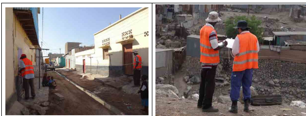
Figure 47 Technology Transfer (Left: Road width measurement; Right: Verification of planimetric features)
