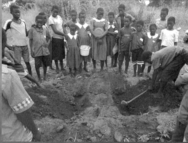
'seven-four' group digging thiers
