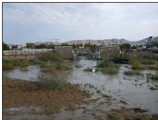
Figure 2 Wastewater discharge into QNR
