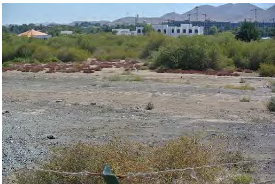
Construction site of QNR
