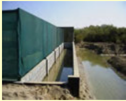
Nursery for seedling production with tidal irrigation system (constructed on 2001)
