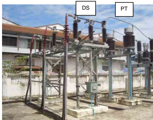
Figure 2-17: 66kV DS (with ES)
