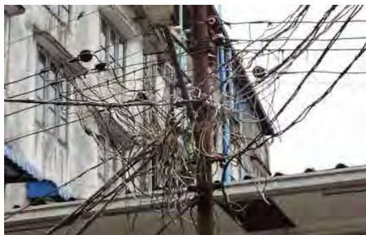
Figure 2-21: Service wire connection in a random manner
