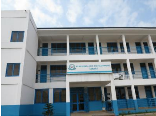
CSTC New Building (Since June 2013)
