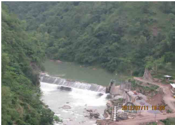
Hydropower dam under construction at Tallo Galyan
