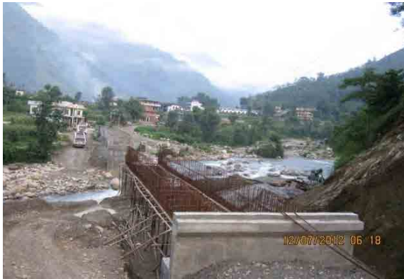
Constructing Bridge On Majuwa Khola(
