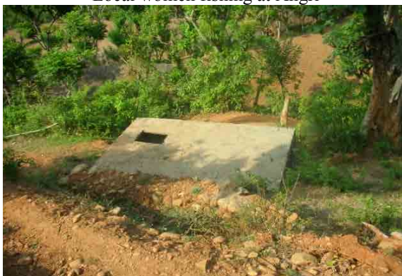
Newly constructed water tank at Damar
