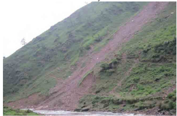
Landslide at Sakala
