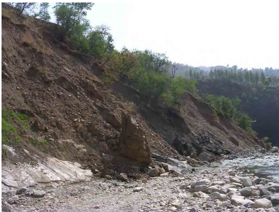
Figure 1.11: Landslide along the Dhansi Khola, at location 079. View to NE.
