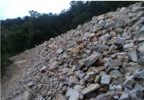
Land slide site near Rabuwa
