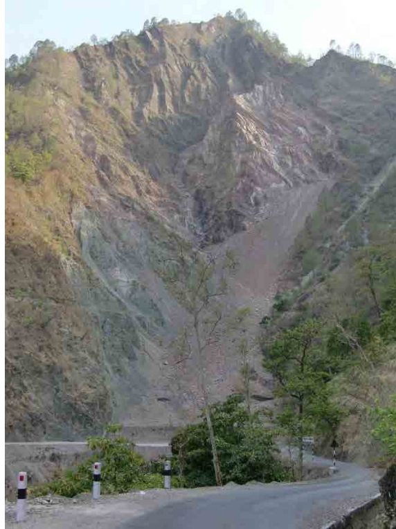
Figure 1.11: Rock slides at pink quartzite and purple shale observed at road section near the village of Gyakhora, near waypoint NAU052. View to SW.
