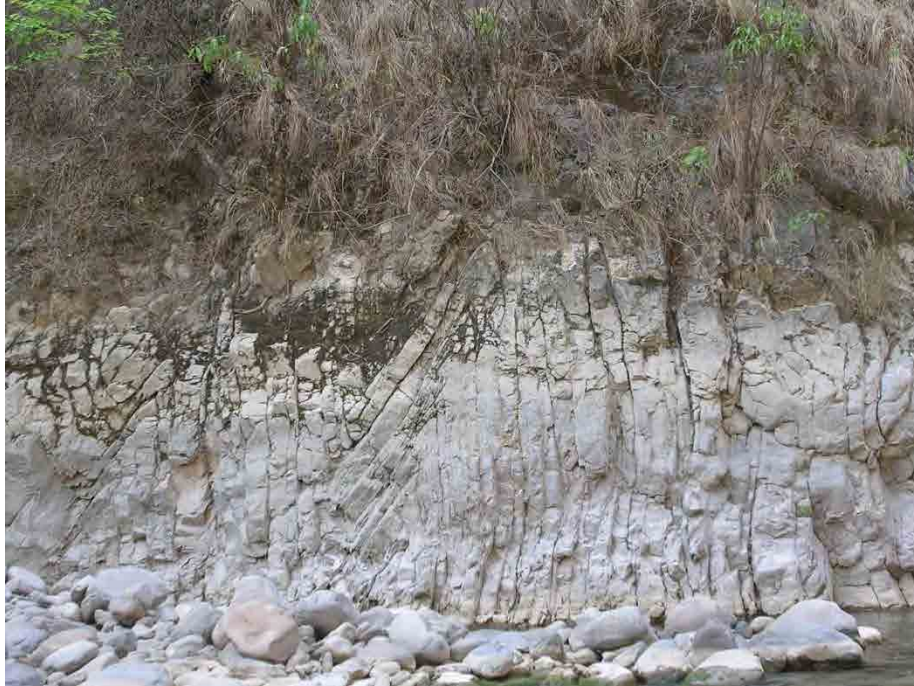
Figure 1.5: Folded rock downstream of the dam site at location 094. View to SE.
