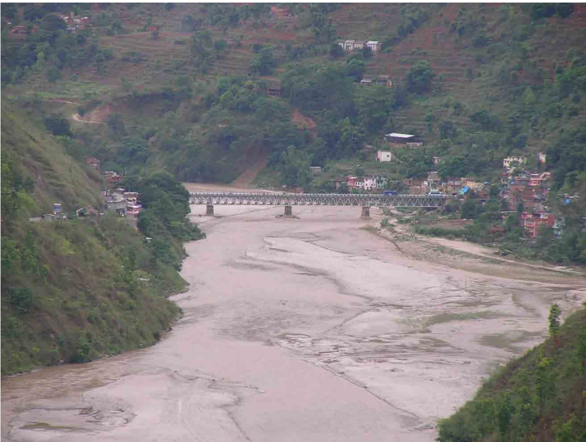
China Bridge of Araniko Highway in Sun Koshi No. 3 Reservoir Area
