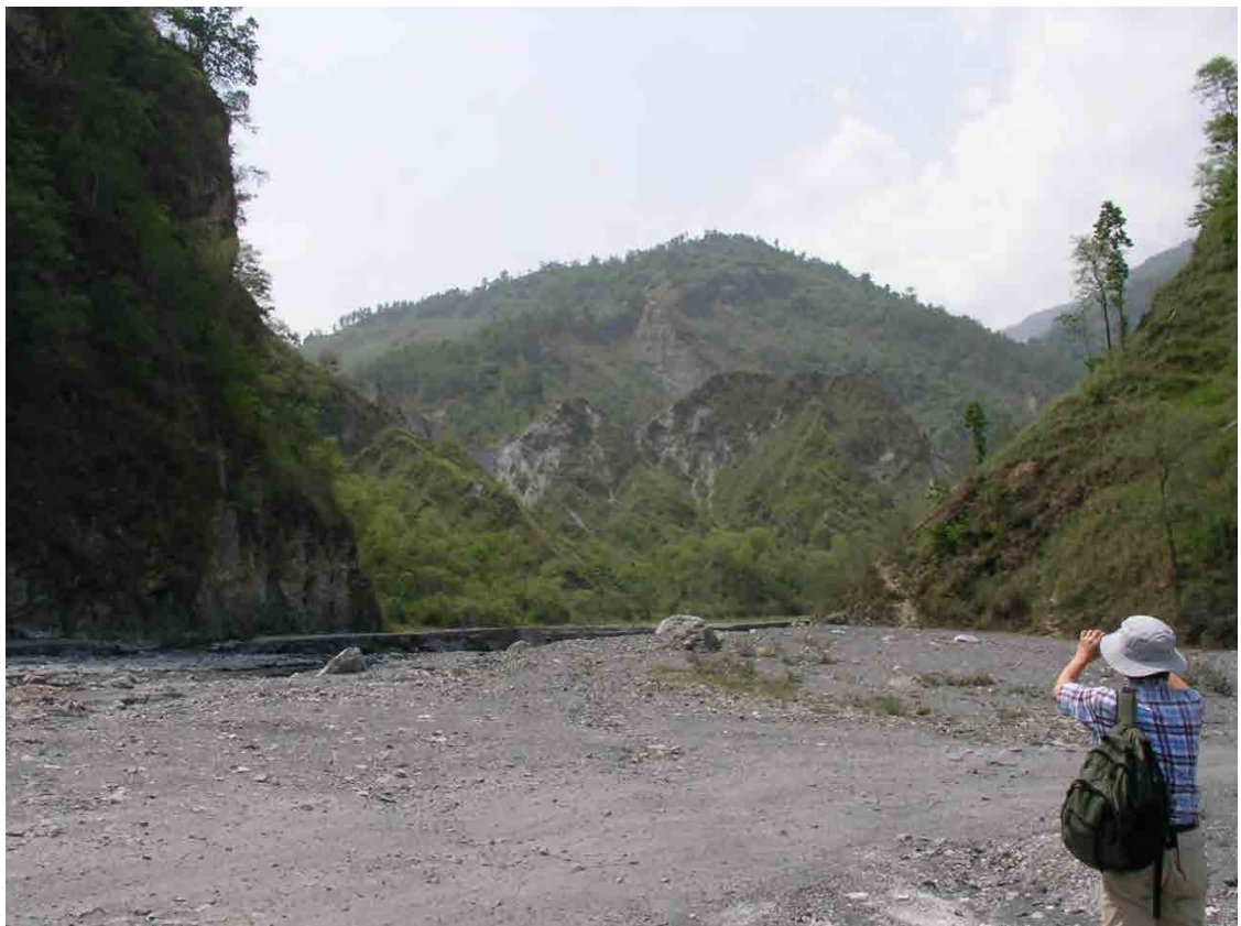
Land Slide Area in Lower Badigad Reservoir Area
