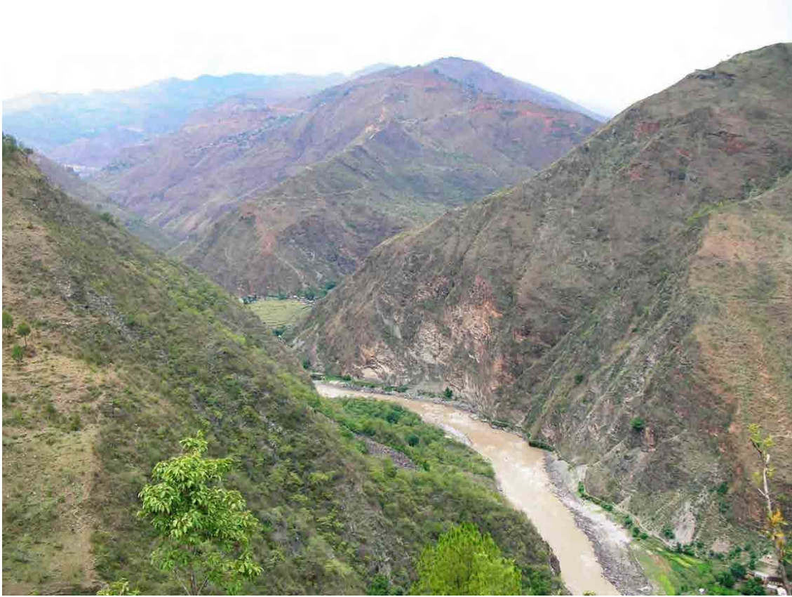
Sun Koshi No. 3 Dam Site View from Downstream
