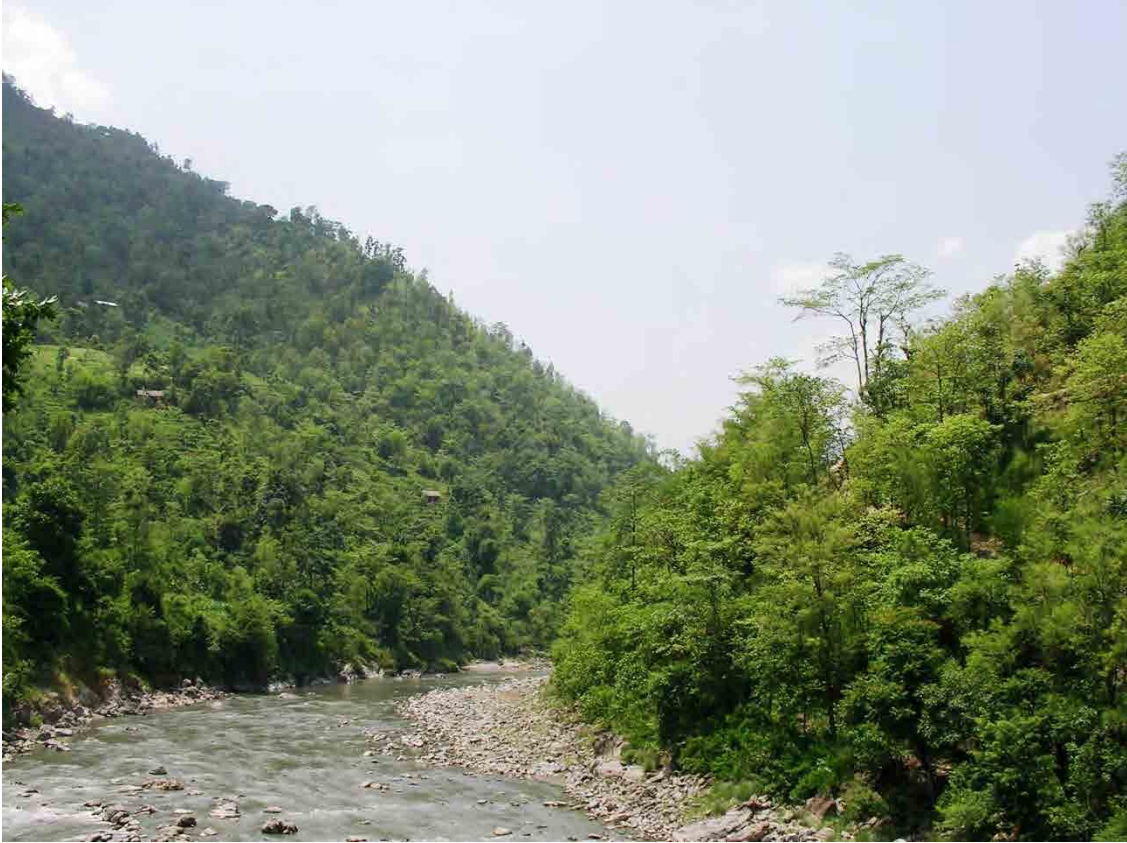
Lower Badigad Dam Site View from Downstream
