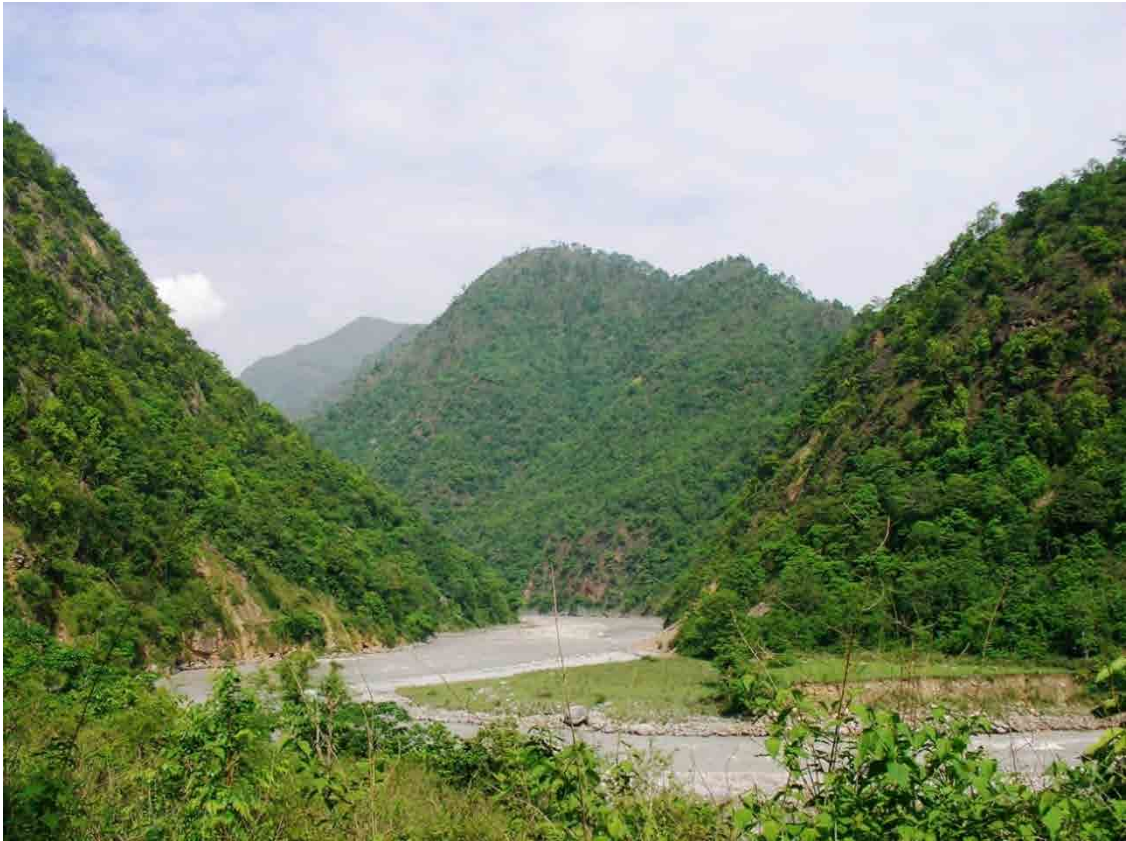
Dudh Koshi Dam Site View from Upstream
