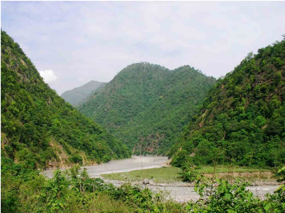
Dudh Koshi Dam Site View from Upstream
