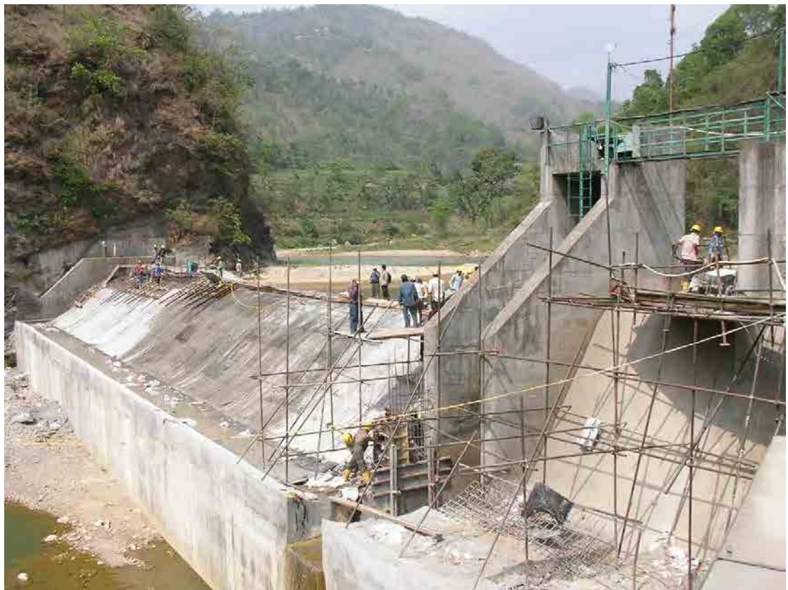
Intake dam of Andhikhola Hydropower Plant (IPP) in Andhi Khola Reservoir Area
