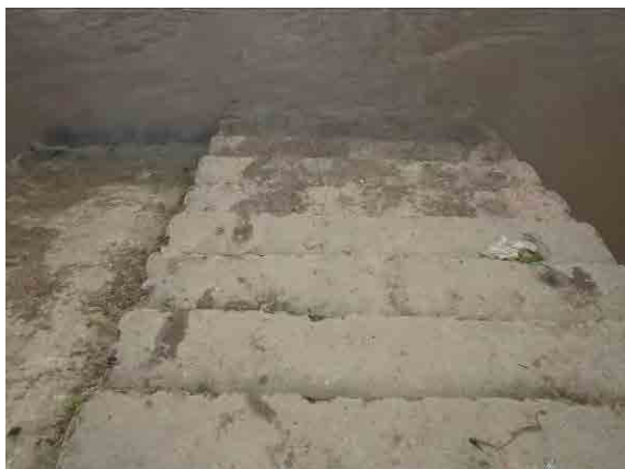
Kalardoba Boat Landing Facility (Zila Boad)* Ghats are mainly Concrete Step type.
