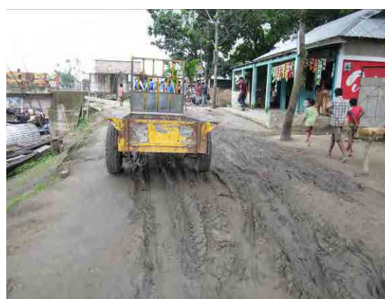
Adarshbazar-Takbazkhani Village Road * (LGED)
