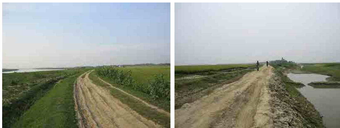
Submersible Embankment in Kairdhar Ratna Scheme
