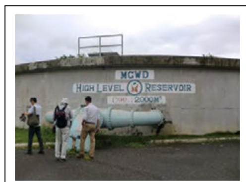
写真-3 Liloan (High Level)配水池
