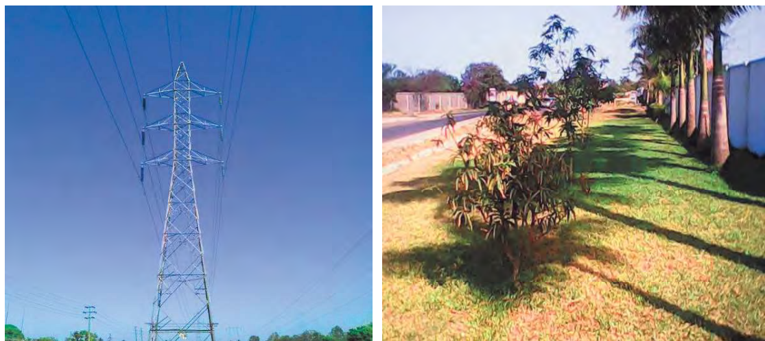
Figure 4.4: Existing way leave from Ubungo to Ilala Substation, the existing towers will be used for replacing lines (Left side) and on rightside the road reserve on Mwaki kibaki road in which the Tegeta to Jangwani line will pass through.
