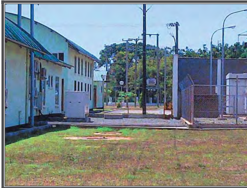
Figure 2.2: Site for the proposed expansion of Msasani S/S
