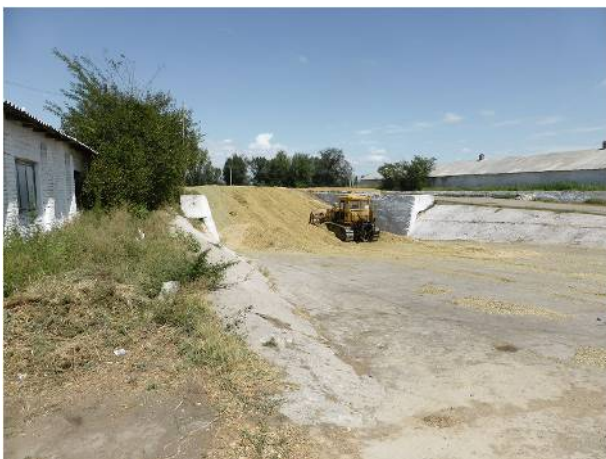
Picture 3-24 Bunker Silo
