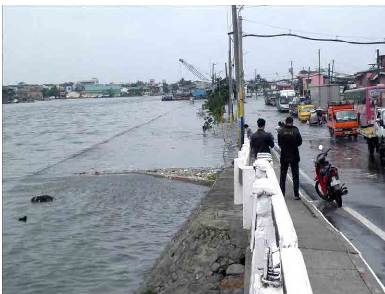
Figure 5.4.1 High Tide on August 2, 2012 at C-4 Bridge of Malabon River Right Bank
