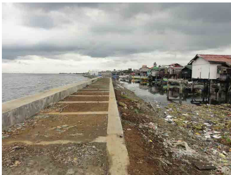
Figure 2.7.3 Constructed Coastal Dike in Navotas City Area
