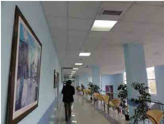
Lightings with magnetic ballast are used → Electronic ballast is more energy saving.
