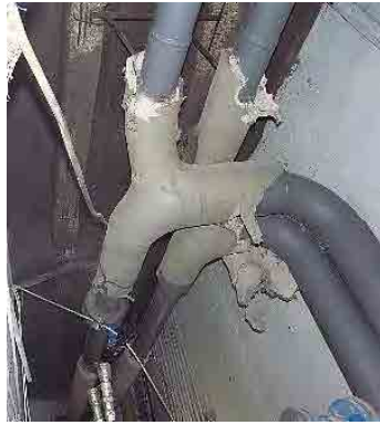
Deteriorated insulation
