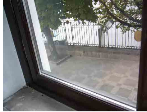
Figure 7-6 Low-e Pair Glasses with Insulated Sash
