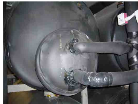
Figure 7-8 Insulation for Hot Water Tank
