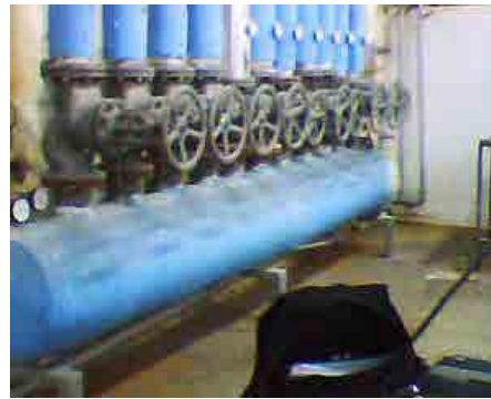
No insulation for valves
