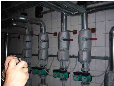
Figure 7-7 Insulation for Valves and Pipes
