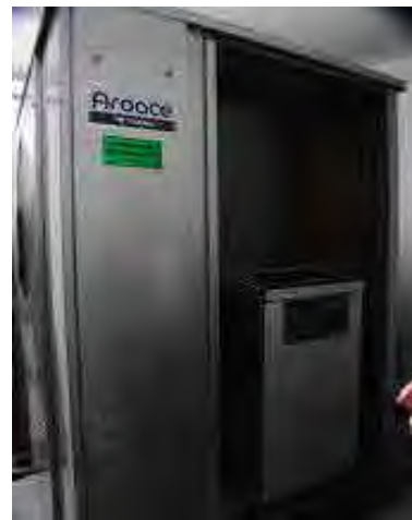
Figure 7-17 Absorption Chiller (YAZAKI)
