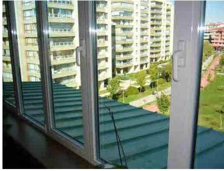
Figure 7-6 Low-e Pair Glasses with Insulated Sash
