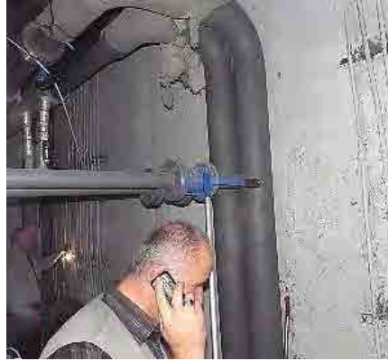
Deteriorated insulation
