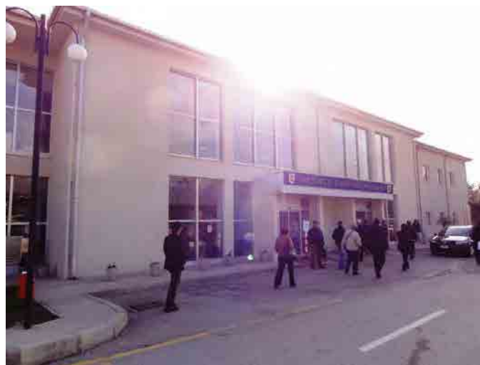
Figure 2.3.2-2 Facade of EM Hospital
