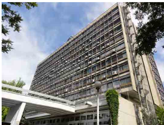
Figure 2.3.2-1 Facade of DSI Buildings
