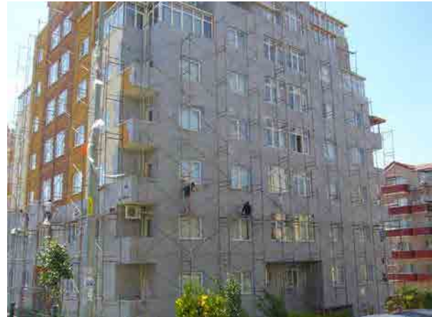
Figure 2.3.3-2 Retrofitting to Add Insulation for Existing Building
