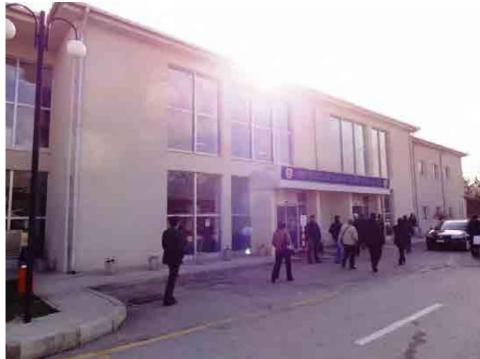
Figure 2.3.2-2 Facade of EM Hospital
