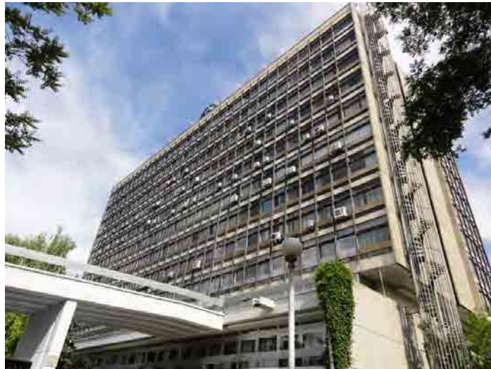
Figure 2.3.2-1 Facade of DSI Buildings
