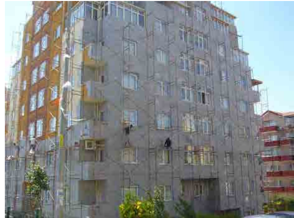
Figure 2.3.3-2 Retrofitting to Add Insulation for Existing Building
