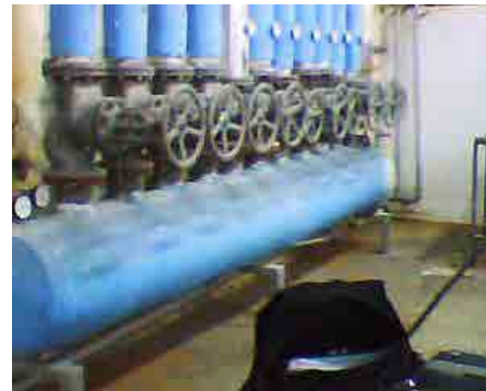
No insulation for valves
