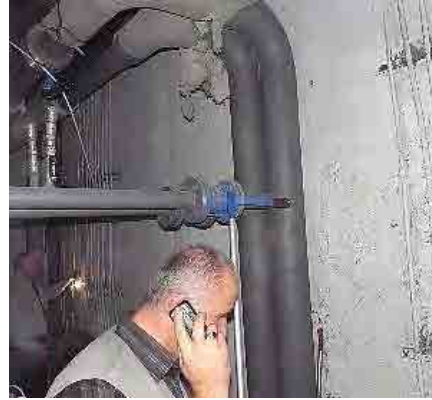
Deteriorated insulation
