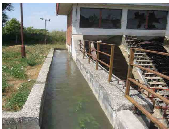
Overflow Channel (in Operation)
