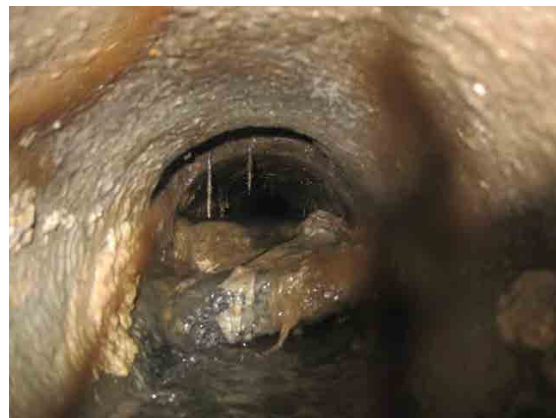
ST-25: Partially Collapsed
