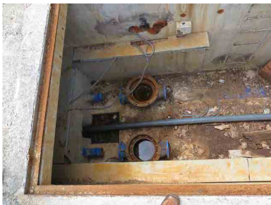
Pump House without Machinery in Elen Kamen PS Source: JICA Study Team
