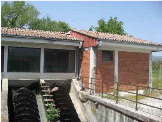
Screw Pump Station
