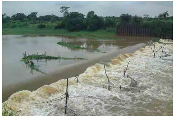
July 2013, Field Survey (Akute Intake and WTP)
