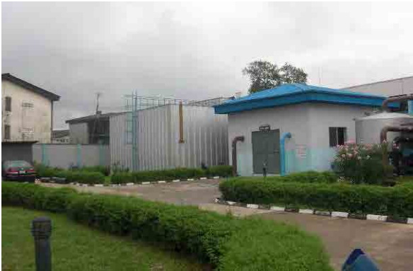
July 2013, Field Survey (Urban Water Supply Facility) Lagos
