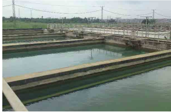
July 2013, Field Survey (Lagos WTP)
