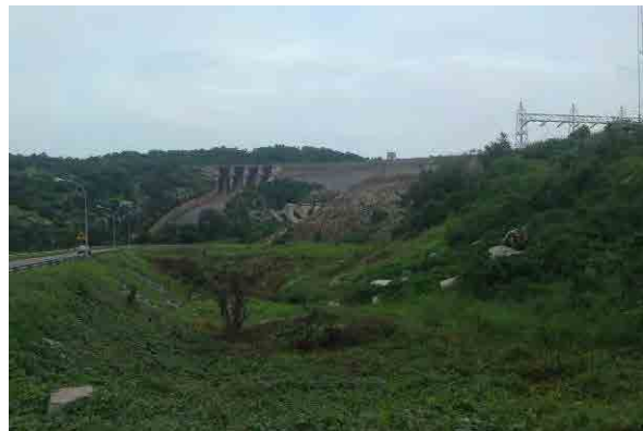
August 2011, Field Survey (Shiroro Dam)
