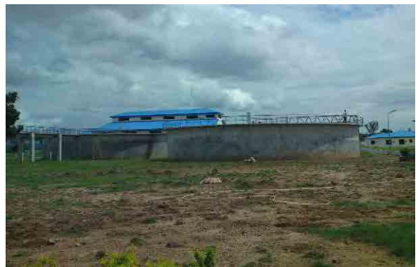
September 2011, Field Survey (WTP in Lokoja)
