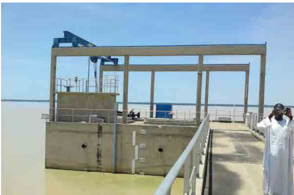
September 2011, Field Survey (Challawa Dam)
