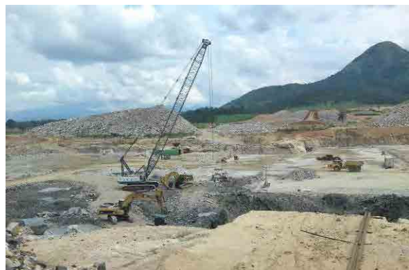
September 2011, Field Survey (Kashimbila Dam Site)
