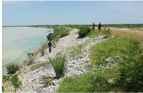
September 2011, Field Survey (Challawa Dam)
