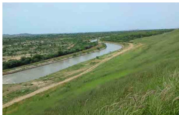
September 2011, Field Survey (Tiga Dam)
