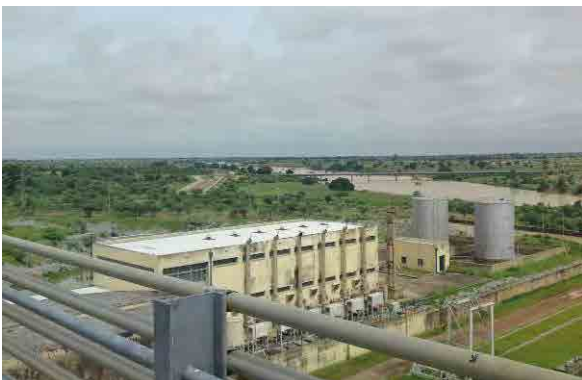
August 2011, Field Survey (Bakolori Dam)
