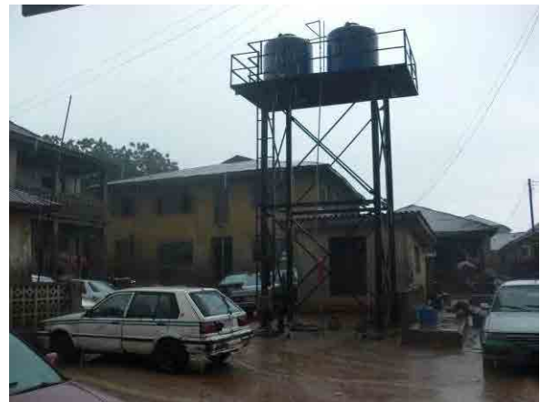
July 2013, Field Survey (Well and Water Supply Facility Ibandan)
