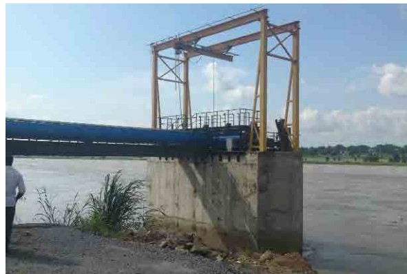
September 2011, Field Survey (WTP in Makarudi)
