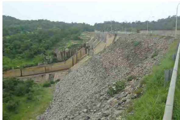
August 2011, Field Survey (Shiroro Dam)
