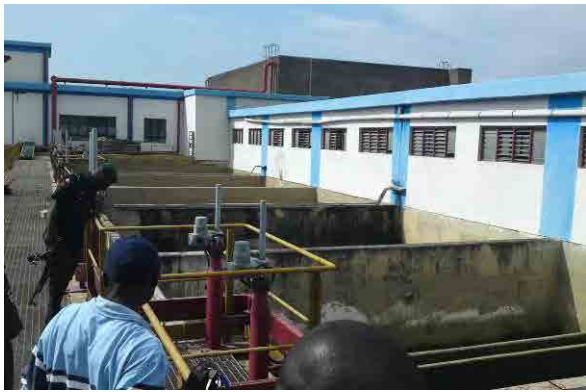
July 2013, Field Survey (Ogun WTP)
