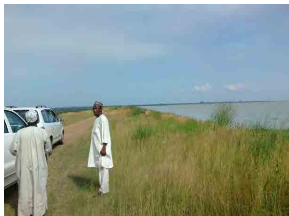
September 2011, Field Survey (Tiga Dam)
