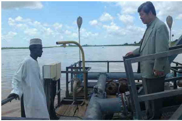
August 2011, Field Survey (Yelwa Intak and WTP)
