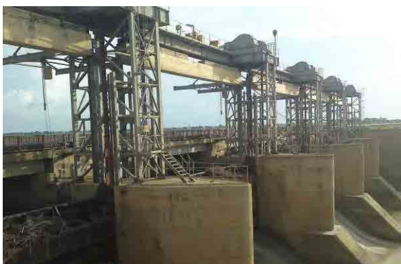
August 2011, Field Survey (Gusau Bridge)
