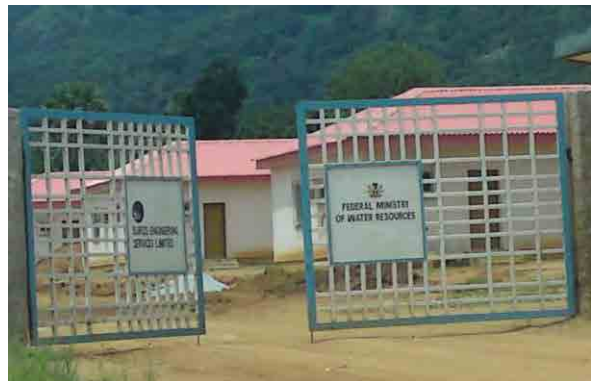
September 2011, Field Survey (Kashimbila Dam Site)
