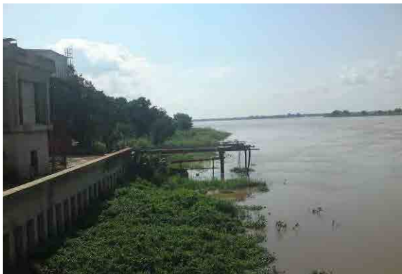
September 2011, Field Survey (WTP in Makarudi)
