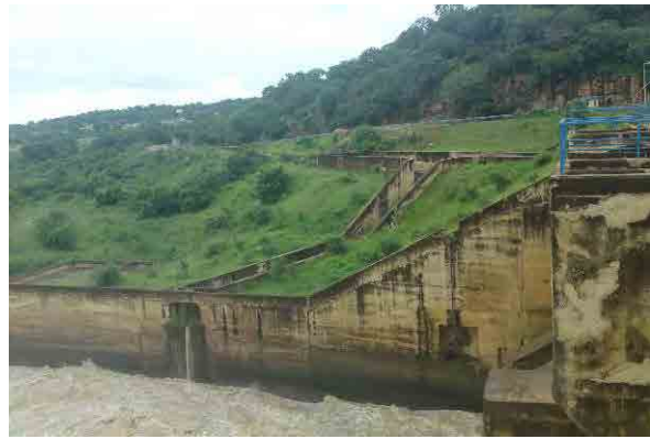
September 2011, Field Survey (Kiri Dam)
