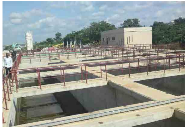
September 2011, Field Survey (WTP in Makarudi)
