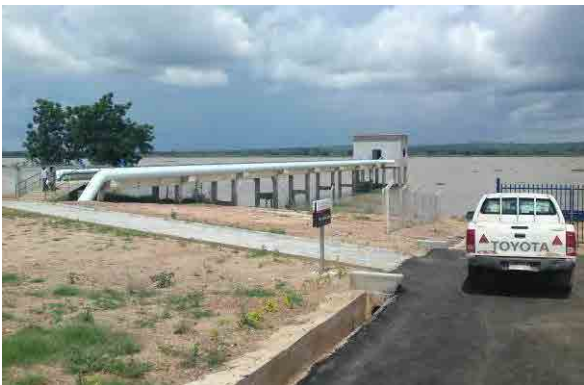
September 2011, Field Survey (WTP in Lokoja)
