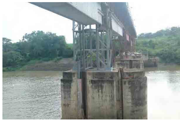
July 2013, Field Survey (Ogun WTP)
