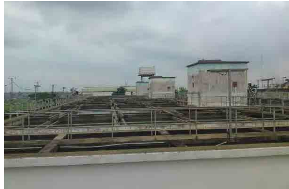
July 2013, Field Survey (Lagos WTP)
