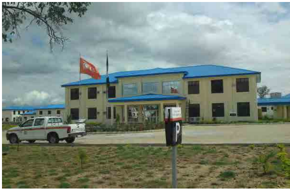
September 2011, Field Survey (WTP in Lokoja)
