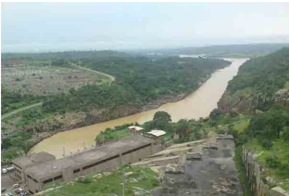
August 2011, Field Survey (Shiroro Dam)
