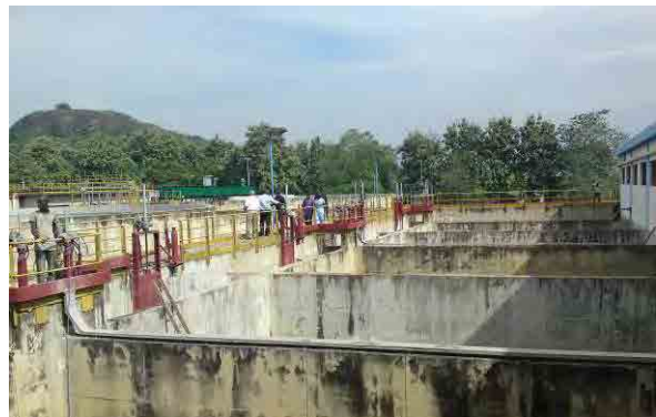
July 2013, Field Survey (Ogun WTP)
