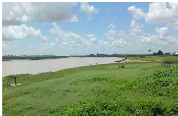
August 2011, Field Survey (Yelwa Intak and WTP)
