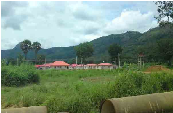
September 2011, Field Survey (Kashimbila Dam Site)
