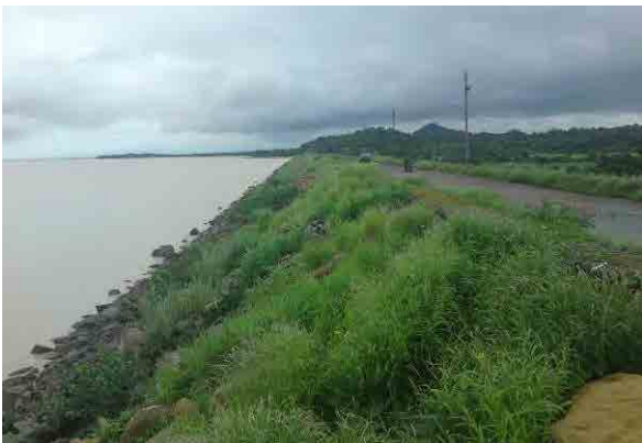
September 2011, Field Survey (Kiri Dam)
