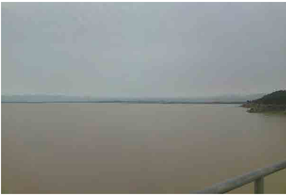
August 2011, Field Survey (Shiroro Dam)
