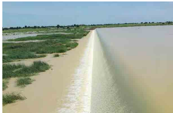
September 2011, Field Survey (Challawa Dam)
