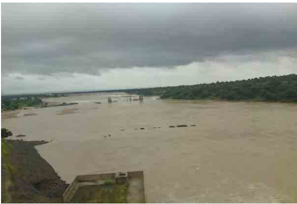
September 2011, Field Survey (Kiri Dam)
