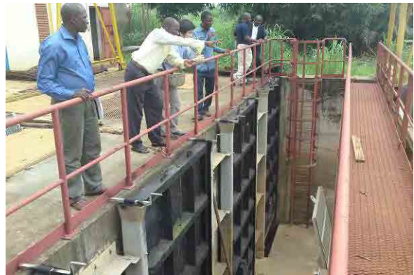
July 2013, Field Survey (Akute Intake and WTP)
