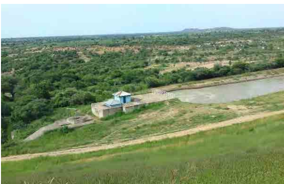
September 2011, Field Survey (Tiga Dam)
