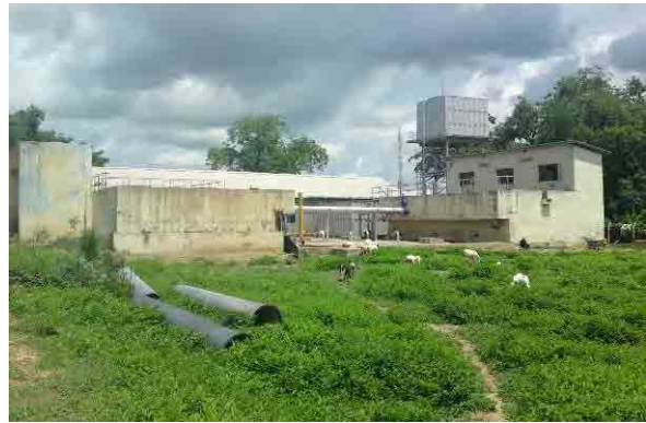
August 2011, Field Survey (Yelwa Intak and WTP)
