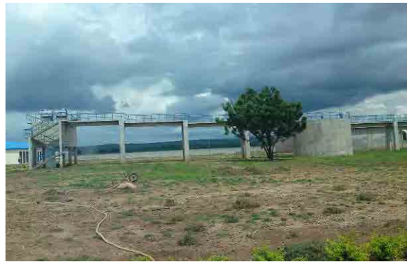
September 2011, Field Survey (WTP in Lokoja)
