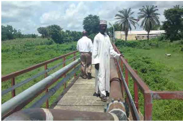
August 2011, Field Survey (Yelwa Intak and WTP)
