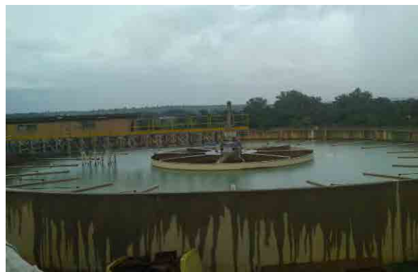
August 2011, Field Survey (WTP in Sokoto)
