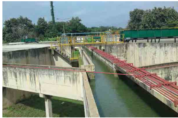
July 2013, Field Survey (Ogun WTP)
