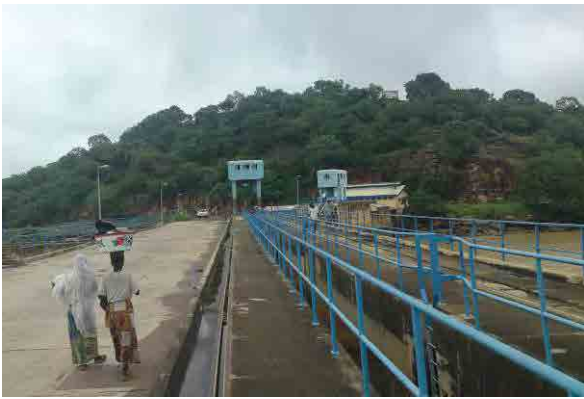
September 2011, Field Survey (Kiri Dam)
