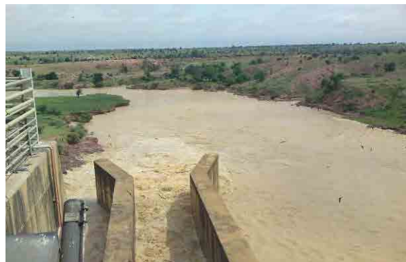
August 2011, Field Survey (Bakolori Dam)
