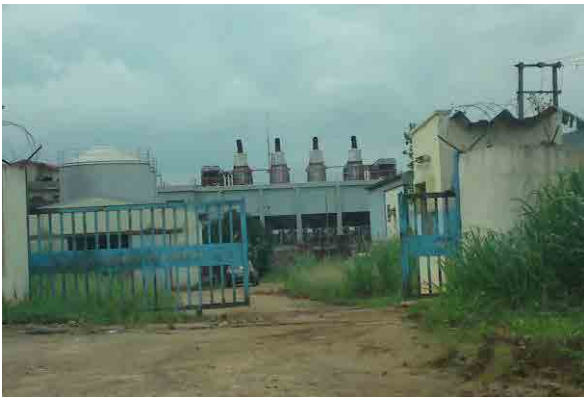
July 2013, Field Survey (Akute Intake and WTP)
