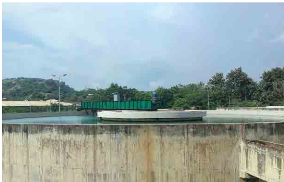
July 2013, Field Survey (Ogun WTP)
