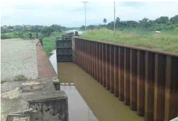
July 2013, Field Survey (Akute Intake and WTP)
