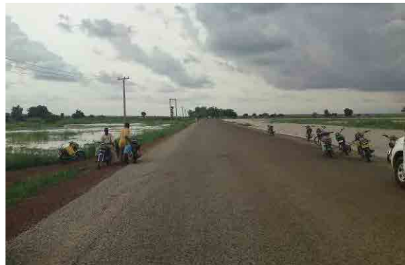
August 2011, Field Survey (Wurno Irrigation Project)
