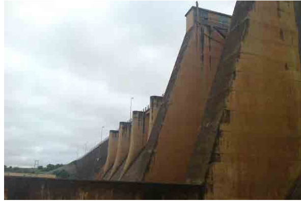
August 2011, Field Survey (Bakolori Dam)
