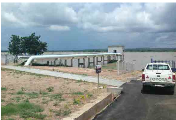
September 2011, Field Survey (Lokoja WTP)
