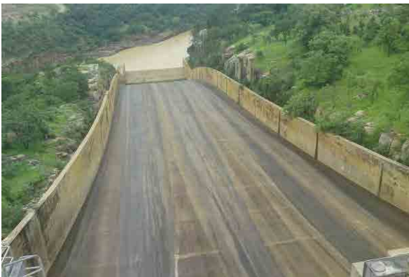
August 2011, Field Survey (Shiroro Dam)
