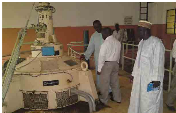
August 2011, Field Survey (Bakolori Dam)
