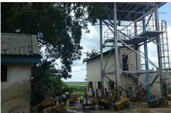
August 2011, Field Survey (Yelwa Intak and WTP)
