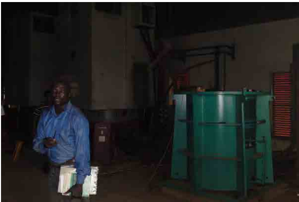
July 2013, Field Survey (Akute Intake and WTP)
