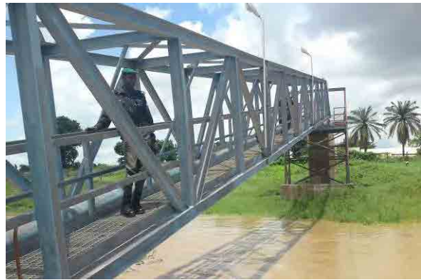
August 2011, Field Survey (Yelwa Intak and WTP)
