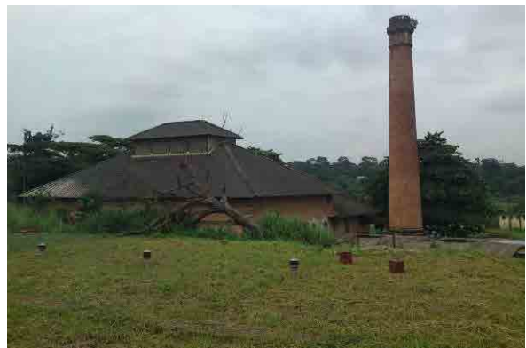
July 2013, Field Survey (Akute Intake and WTP)
