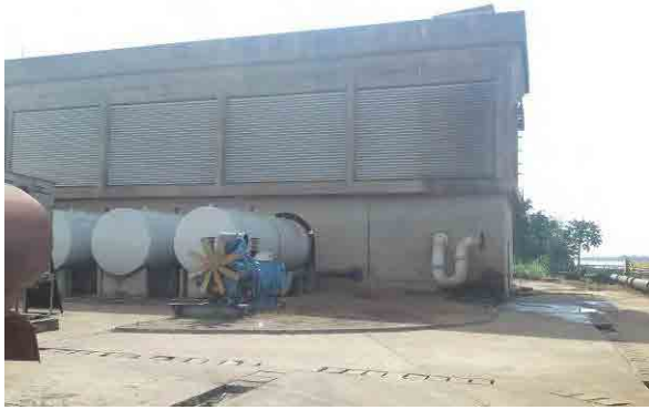
September 2011, Field Survey (WTP in Makarudi)
