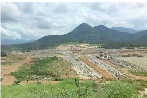
September 2011, Field Survey (Kashimbila Dam Site)
