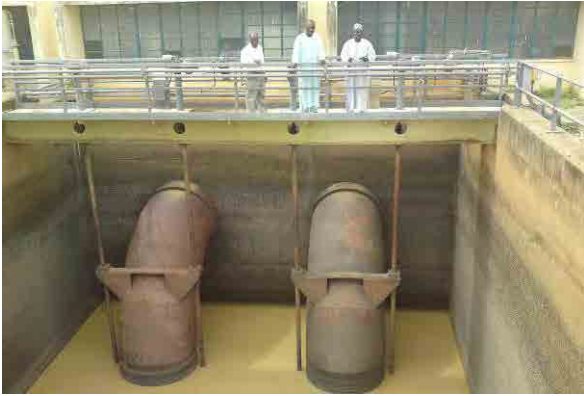
August 2011, Field Survey (Bakolori Dam)
