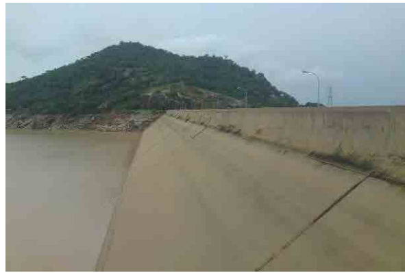
August 2011, Field Survey (Shiroro Dam)
