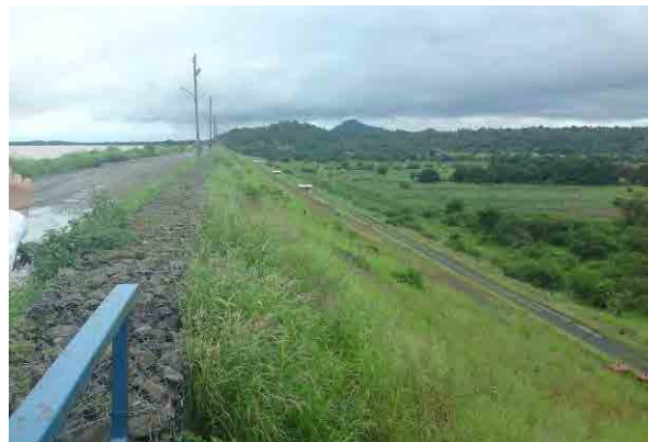
September 2011, Field Survey (Kiri Dam)
