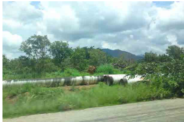
September 2011, Field Survey (Kashimbila Dam Site)
