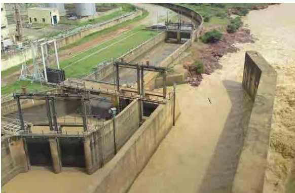
August 2011, Field Survey (Bakolori Dam)
