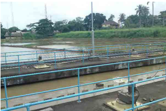
July 2013, Field Survey (Akute Intake and WTP)
