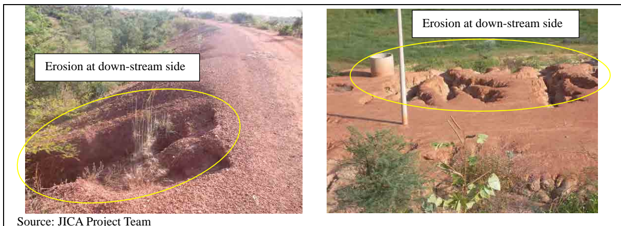
Photo 8-2 Erosions of Gari Dam Body
