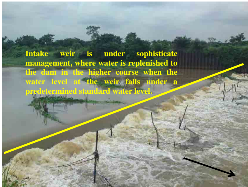
Photo 8-1 Intake Weir in the Downstream in Ogun-Oshun Basin (managed with a standard water level to request replenishment of water to the dam)
