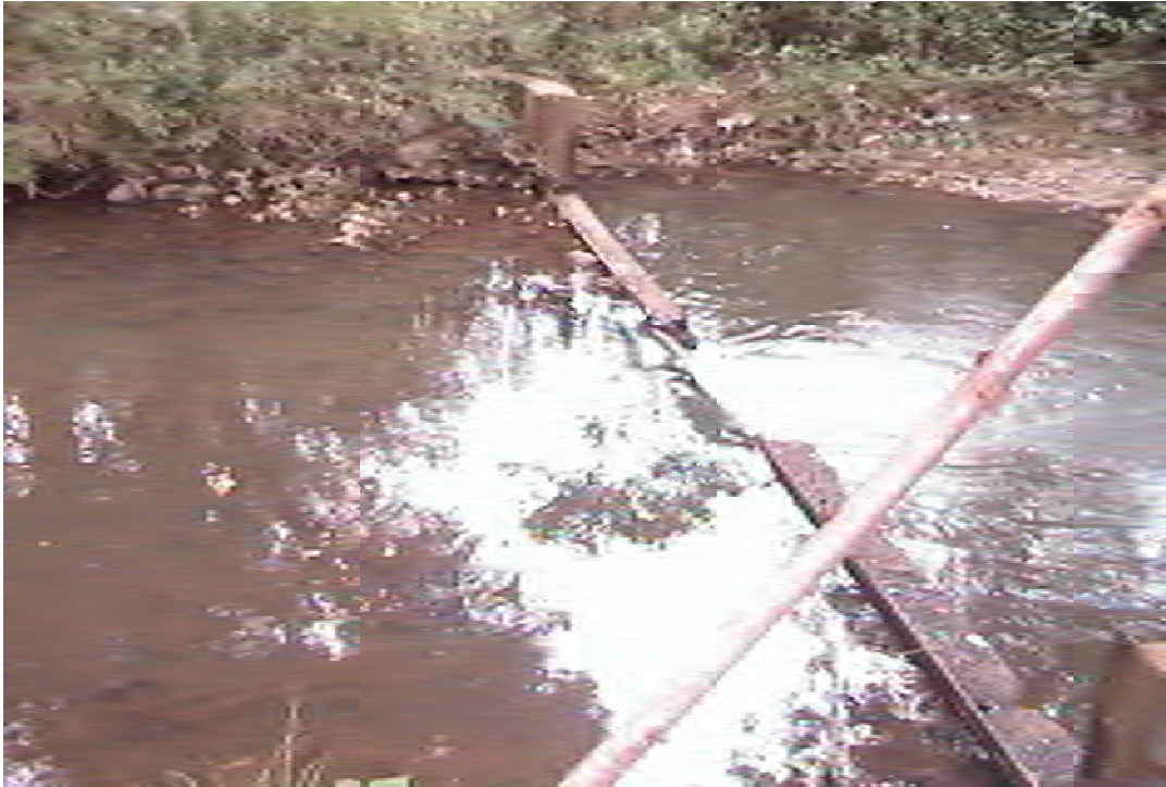
Figure 7: Combined V-Notch and Broadcrested weir (Compound weir)
