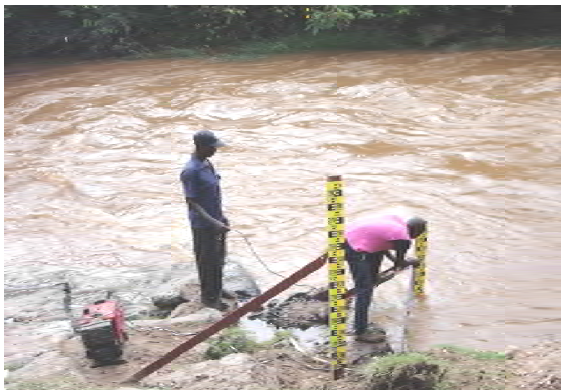
Figure 8: Installation of manual vertical gauges on metal posts
