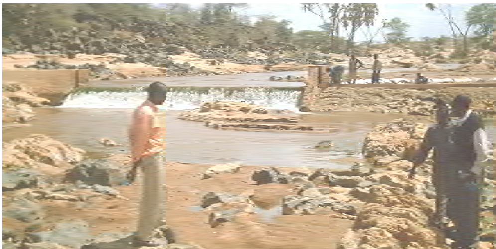
Figure 5: Broad-crested weir
