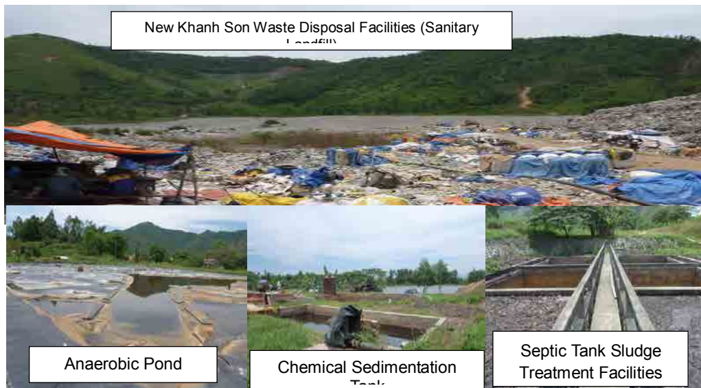
Figure 3.19 Khanh Son Waste Disposal Facilities and Leachate Treatment Facilities
