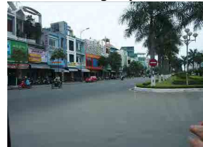
Figure 3.7 Road and Bridge in Da Nang City
