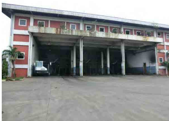
Transfer Station at Sunter
