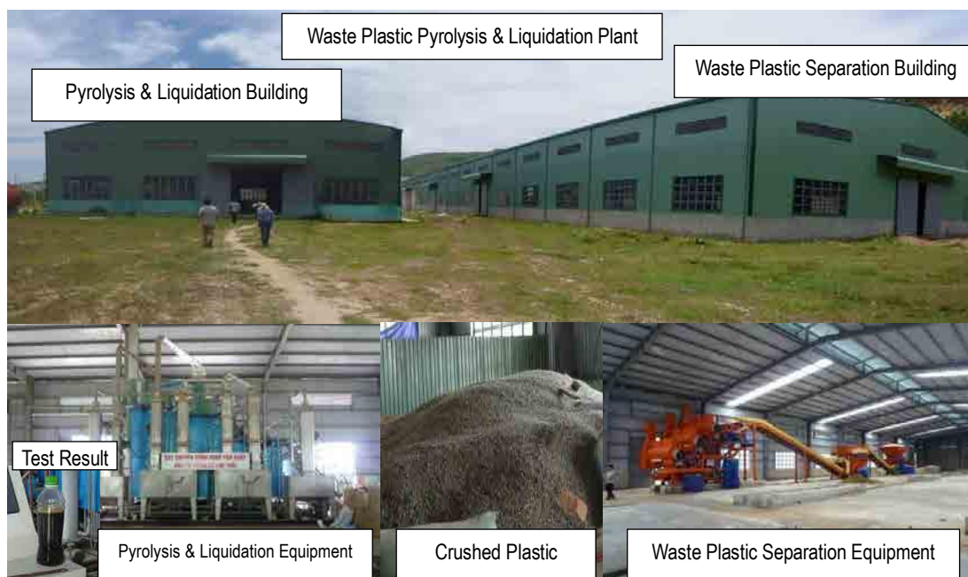
Figure 3.18 Waste Plastic Separation, Pyrolysis and Liquidation Plant in Construction
