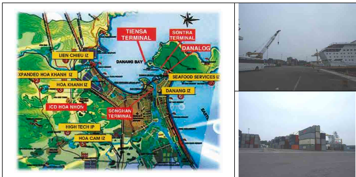
Figure 3.9 Area around Danang Port and photographs of the present state
