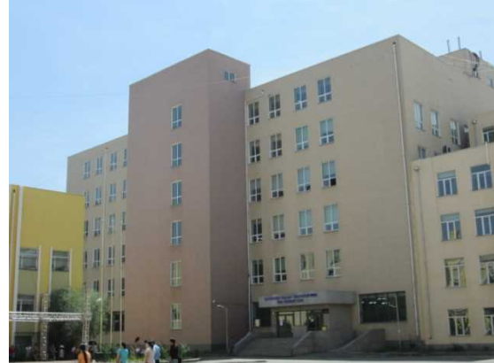
Photograph: Library Building (viewed from the patio)
