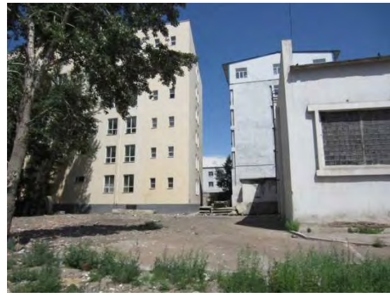
Photograph: Planned building construction site on the MUST campus
