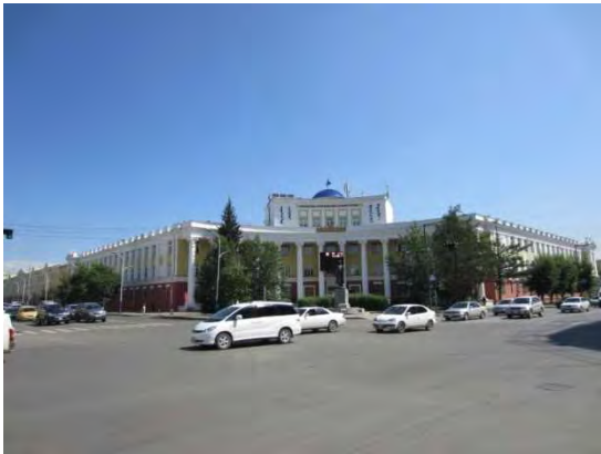
Photograph: Façade of the 1 st Building
