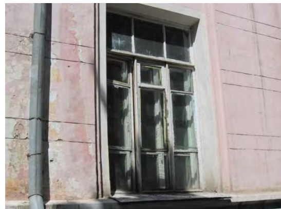
Photograph: A window which has not been renovated (6 th Building, NUM)
