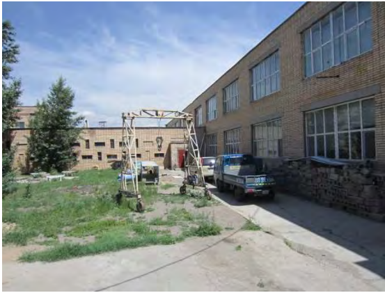
Photograph: Patio, Bridge Building (background) and the 3 rd Building (right)
