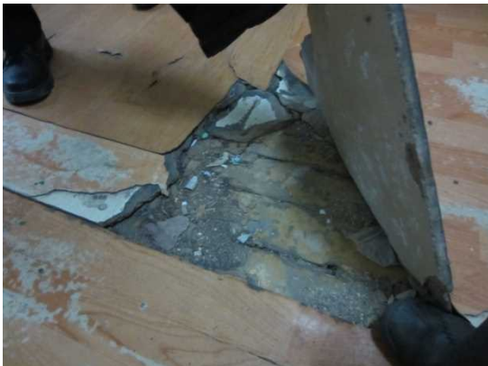
Photograph: A flooring sheet laid over the old floor
