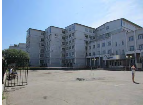
Photograph: The 2 nd Building (viewed from the parking lot)
