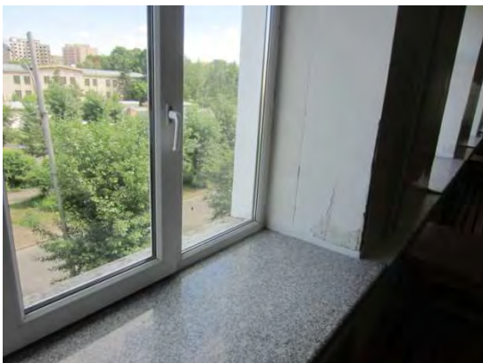
Photograph: A renovated window (2 nd Building, MUST)
