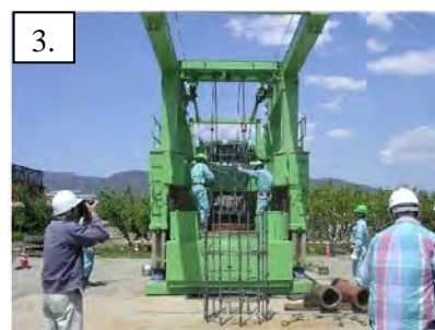
Figure 6.1.2-1 Construction Steps of Additional Pile Foundation (Cast-in-place Concrete Pile)
