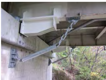
Typical application of steel bracket
