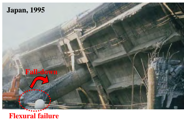
Figure 1.2-1 Flexural Failure of Columns
