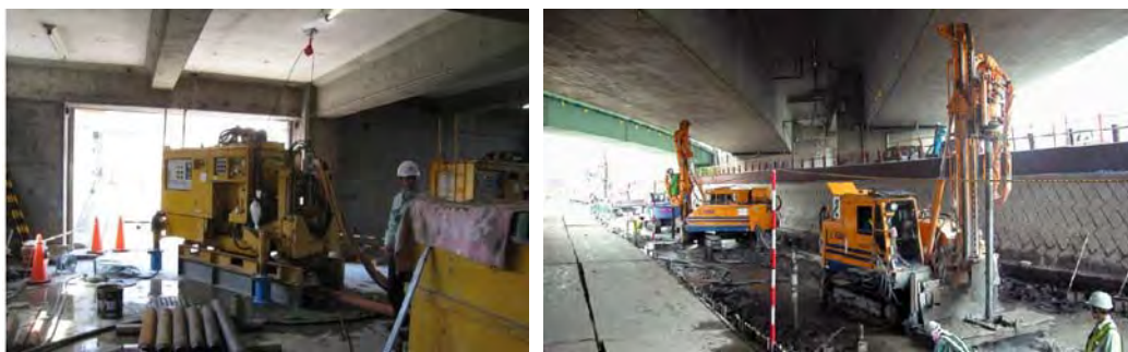
Figure 7.1.3-2 Application Example of Soil Improvement Method under Existing Structures
