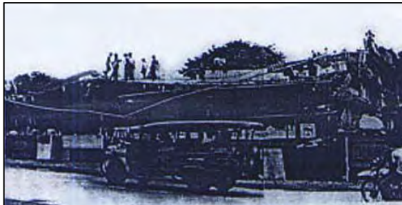
Collapse building due to shear and torsional failure
