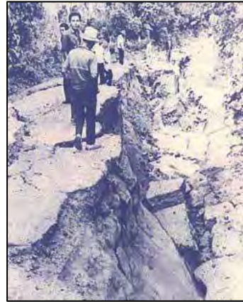
Fissures on road from Casiguran to Barrio Tabas
