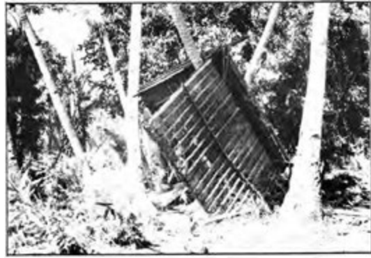
Wall and flooring of nipa hut swept away by tsunami (Brgy. Malaylay, Baco)
