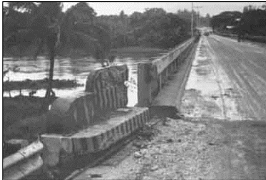
Centerline offset at Tamontaka Bridge
