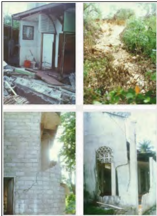
Partial collapse of building; shear cracks
