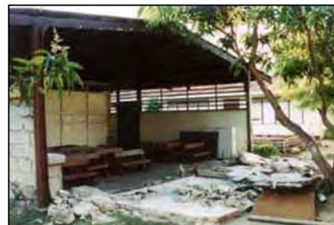
Collapsed concrete wall of a school building in Dimasalang, Masbate.
