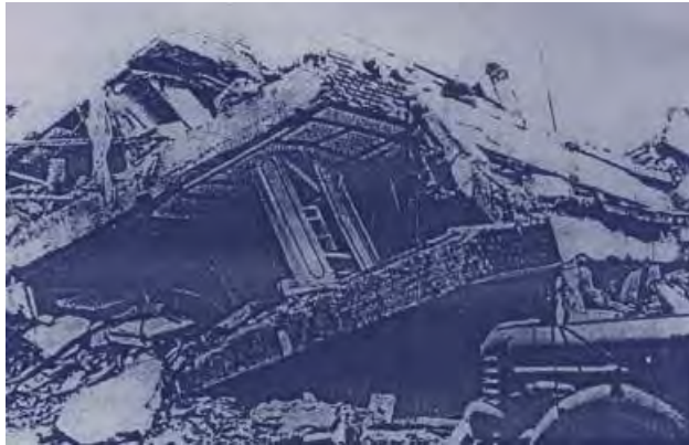
Shear and torsion failure of Denson Building (Laoag City)
