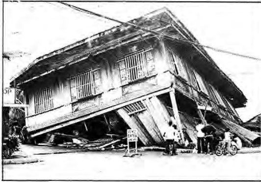
Collapse of old house due to ground shaking (Calapan town proper)
