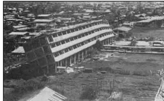
Failure of lower floors at Harvardian College
