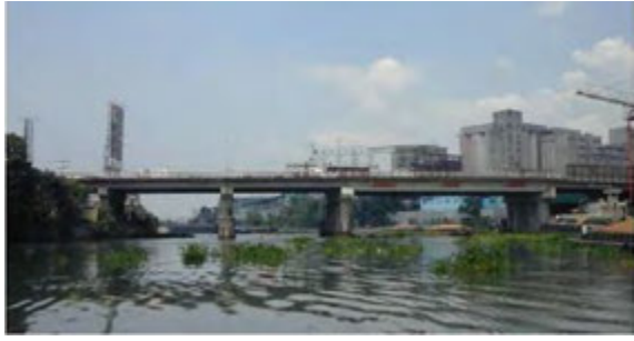
B11 C-5 Bridge
