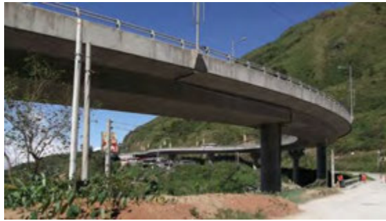
C01 Badiwan Bridge
