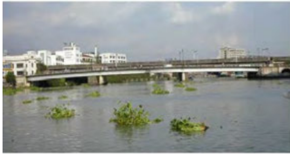
B03 Mc Arthur Bridge
