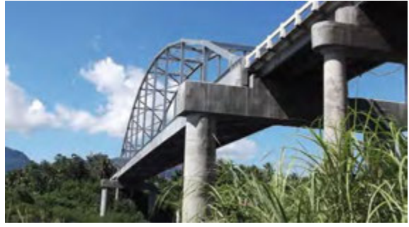
C12 Biliran Bridge
