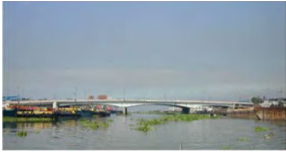
B01 Delpan Bridge
