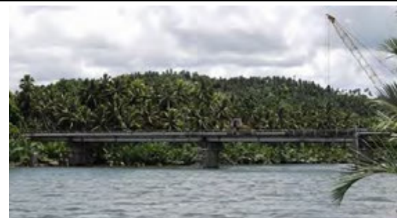
C10 Jibatang Bridge
