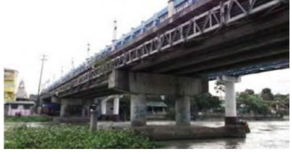
B12 Bambang Bridge
